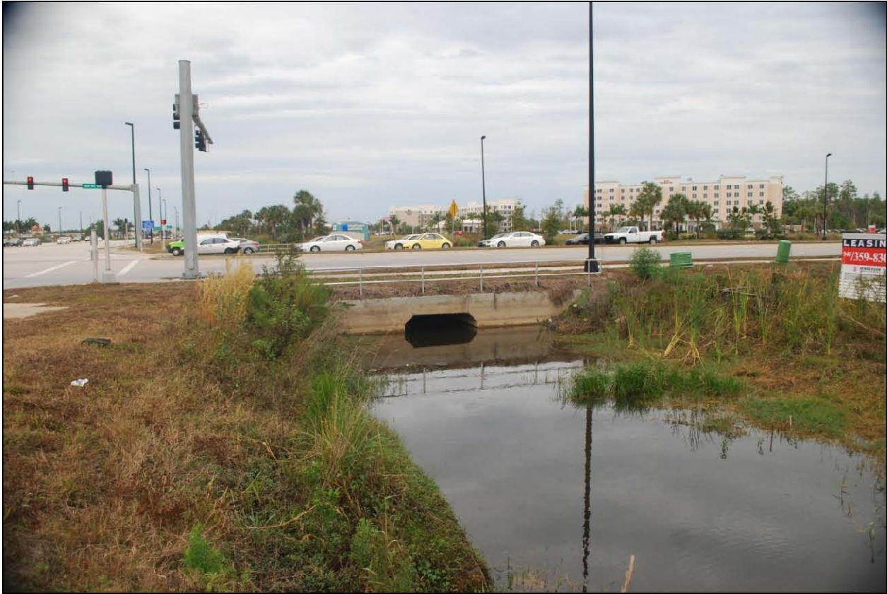
Figure 2.6.1 Existing Box Culvert at North Ditch
