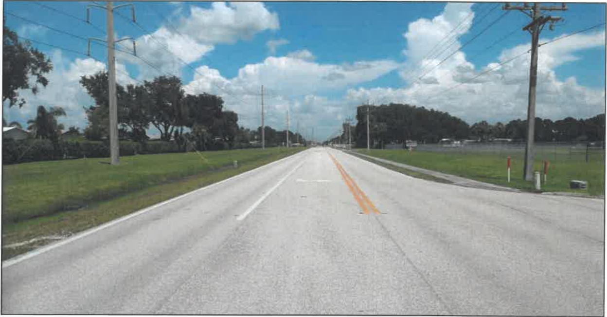
Figure 2-2 - Littleton Road Looking East from Hutto Road
