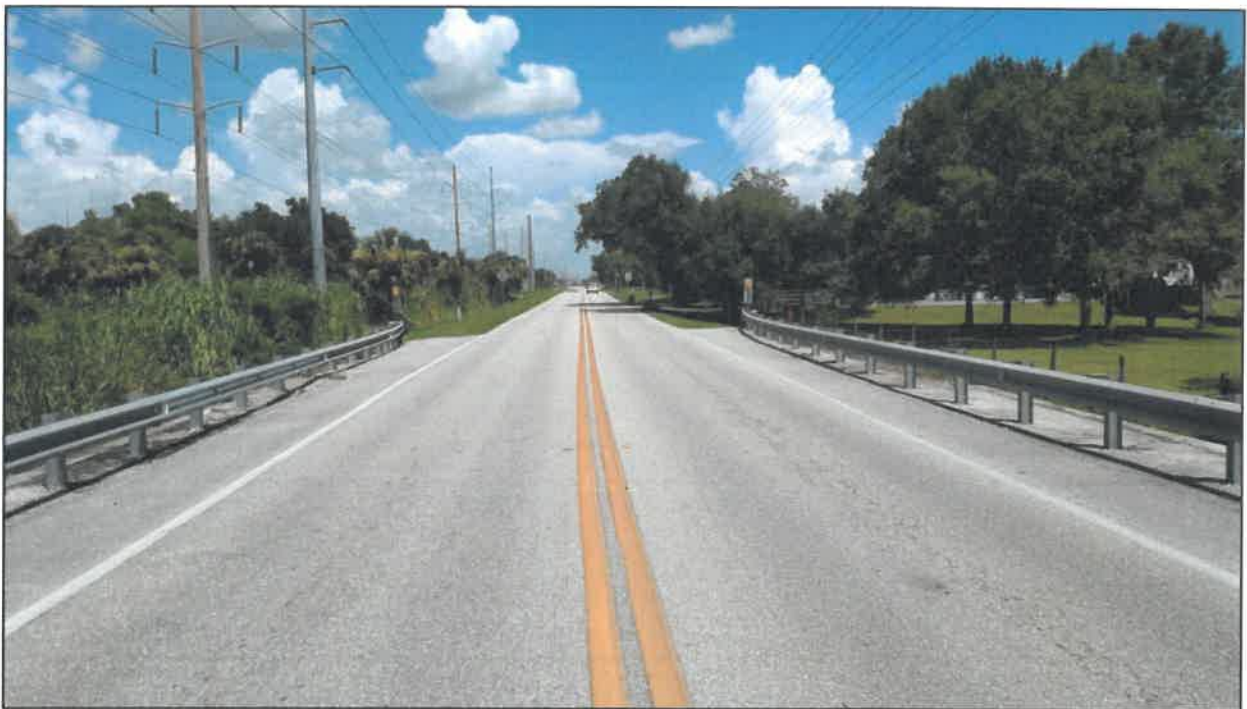
Figure 2-1 - Littleton Road Looking East from Corbett Road
