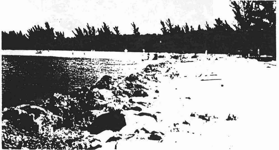
Figure 27A. North end of Bonita Beach showing former inlet site and proximity of new construction. Fig. 27B. Ground photo of area shown in Fig. 27A. Note that there is little to no beach. Fig. 27C. Boulder revetment north of area shown in Fig. 27B. This affords little protection in area of chronic erosion or during storms.
