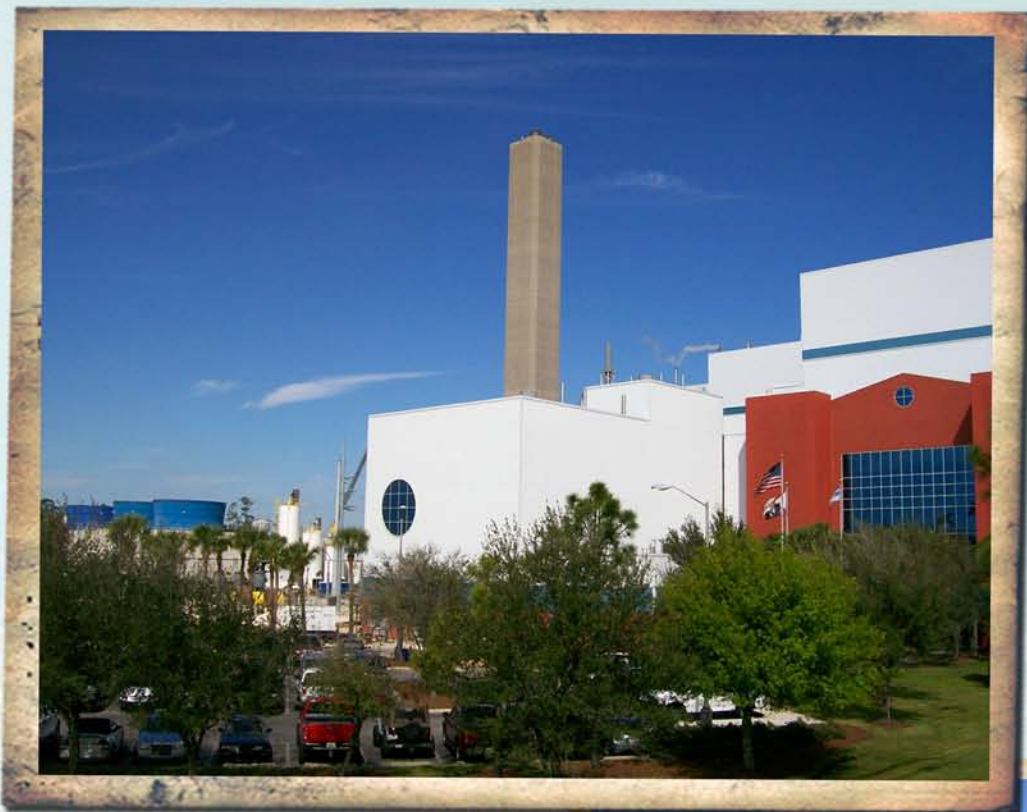
New Combustion Unit
