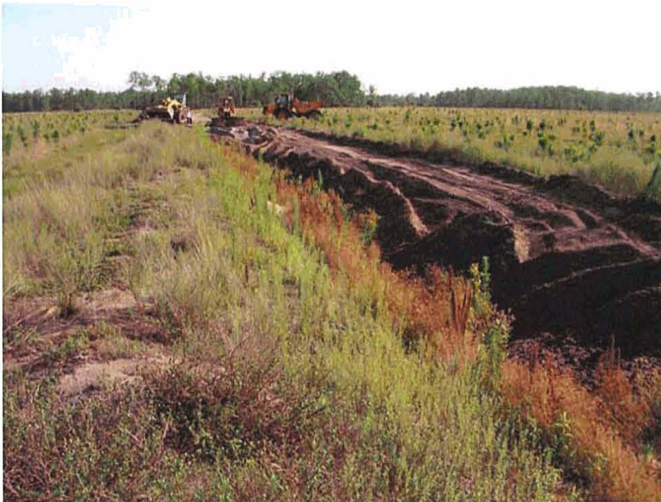
Backfilling agricultural ditches (2008)
