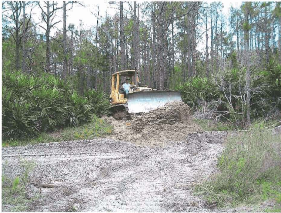
Breaching existing berm to restore sheet flow (2008)
