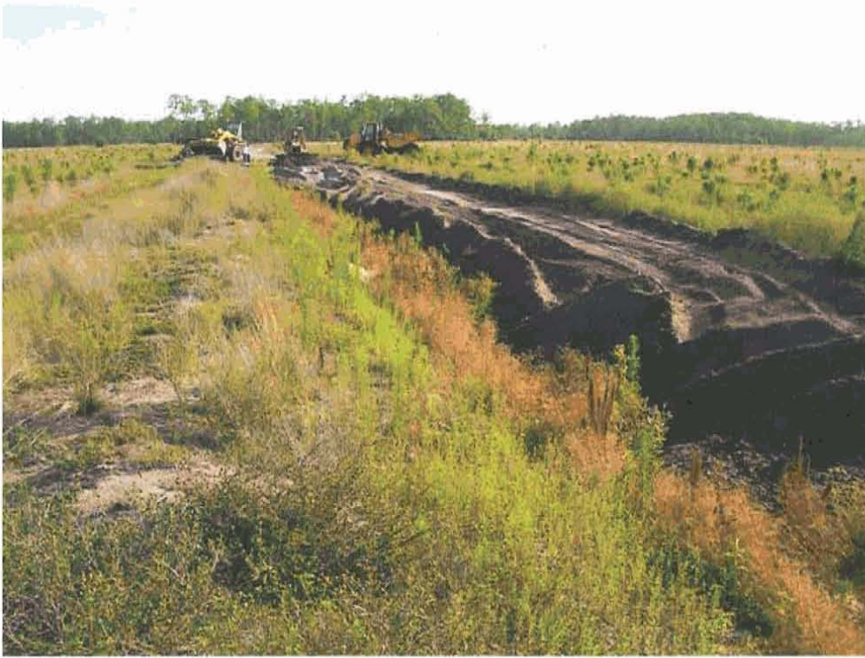
Backfilling agricultural ditches (2008)
