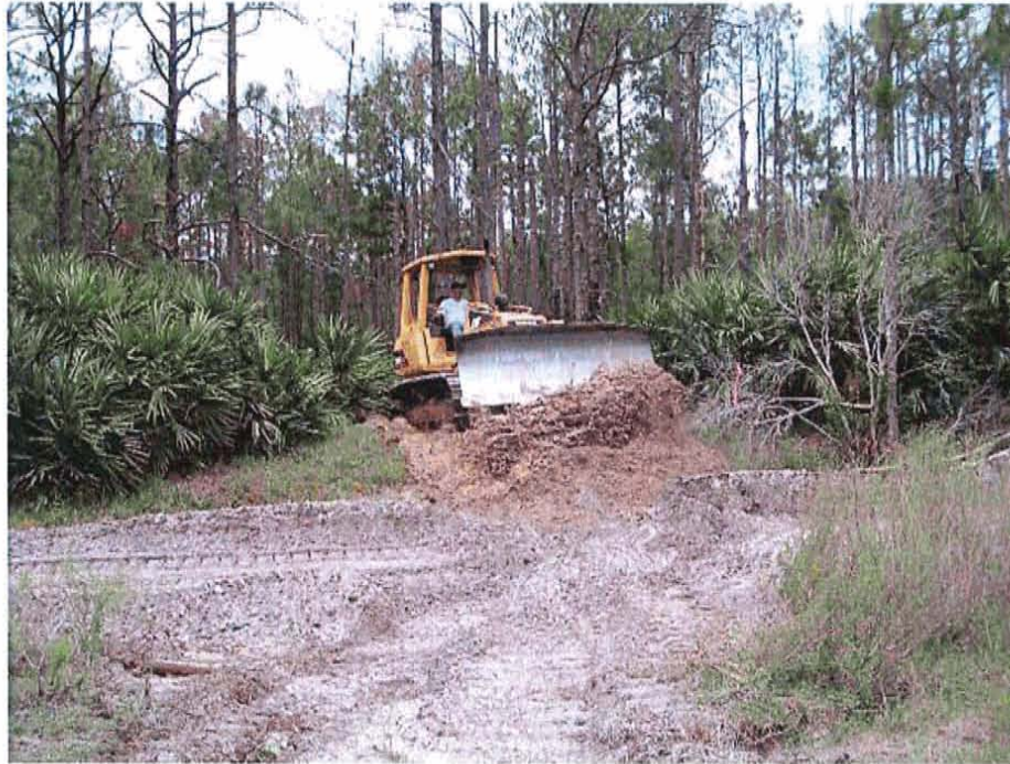
Breaching existing berm to restore sheet flow (2008)
