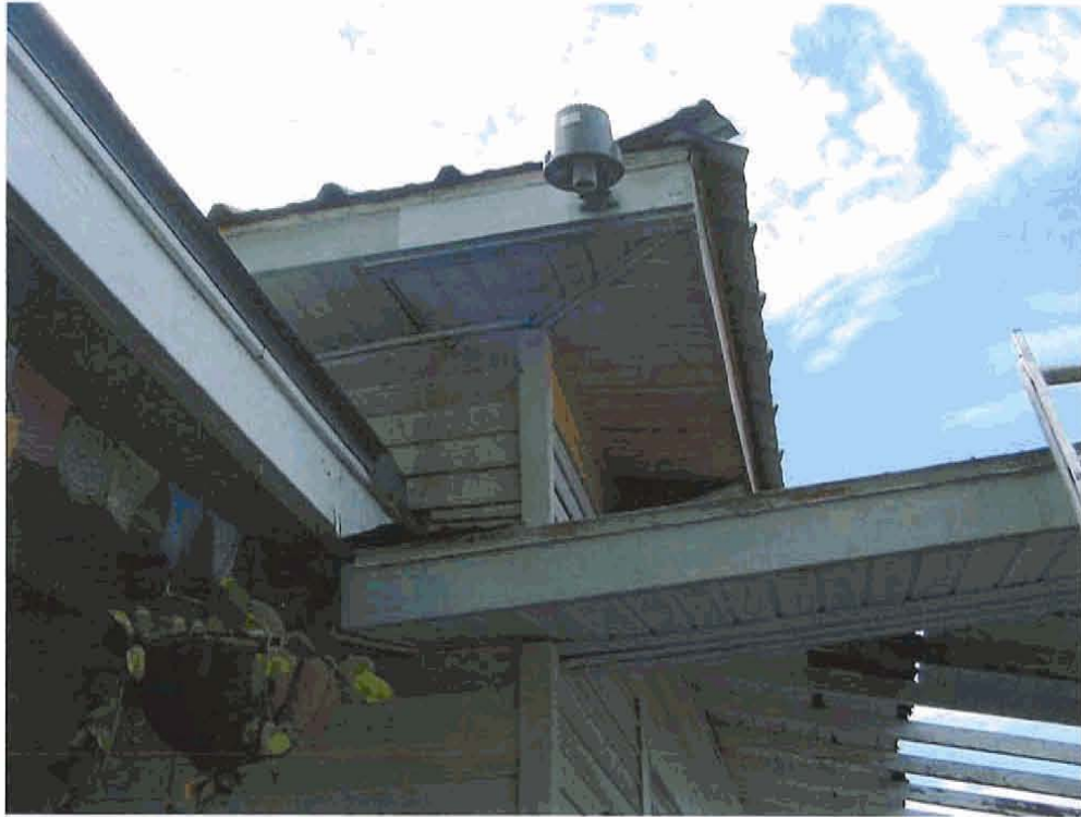
Front porch showing current roof line
