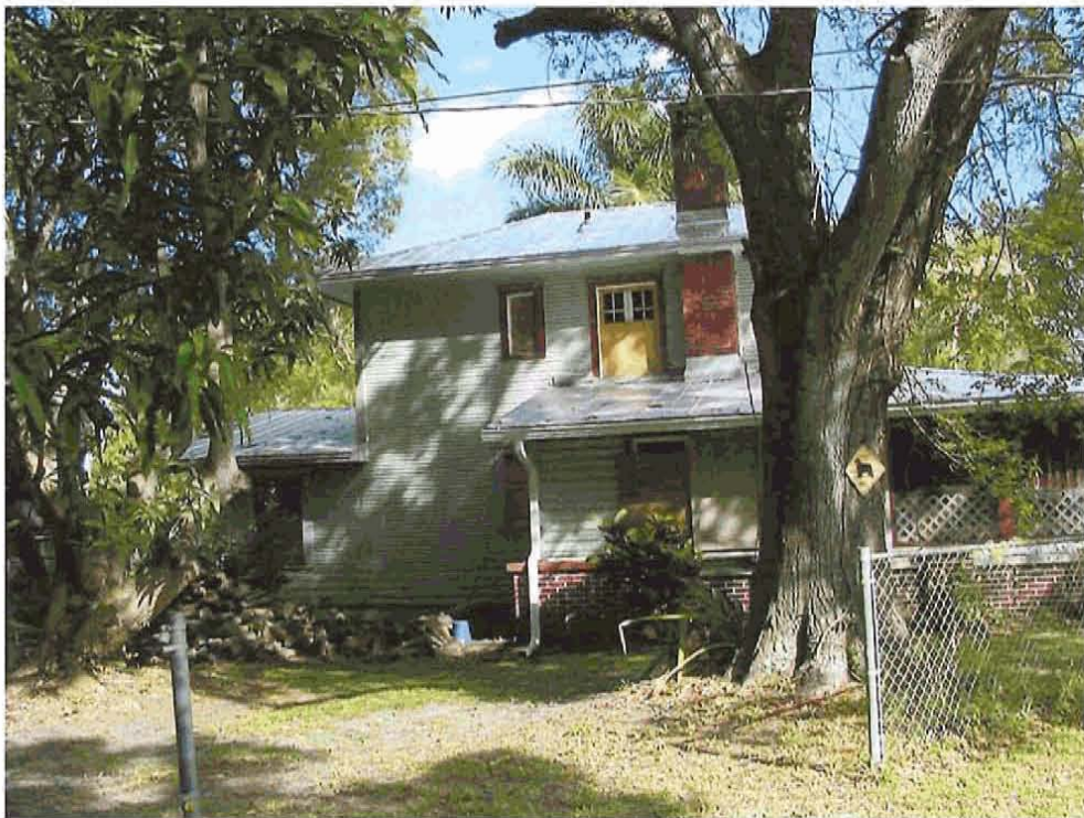
Right (south) elevation seen from Prospect Ave
