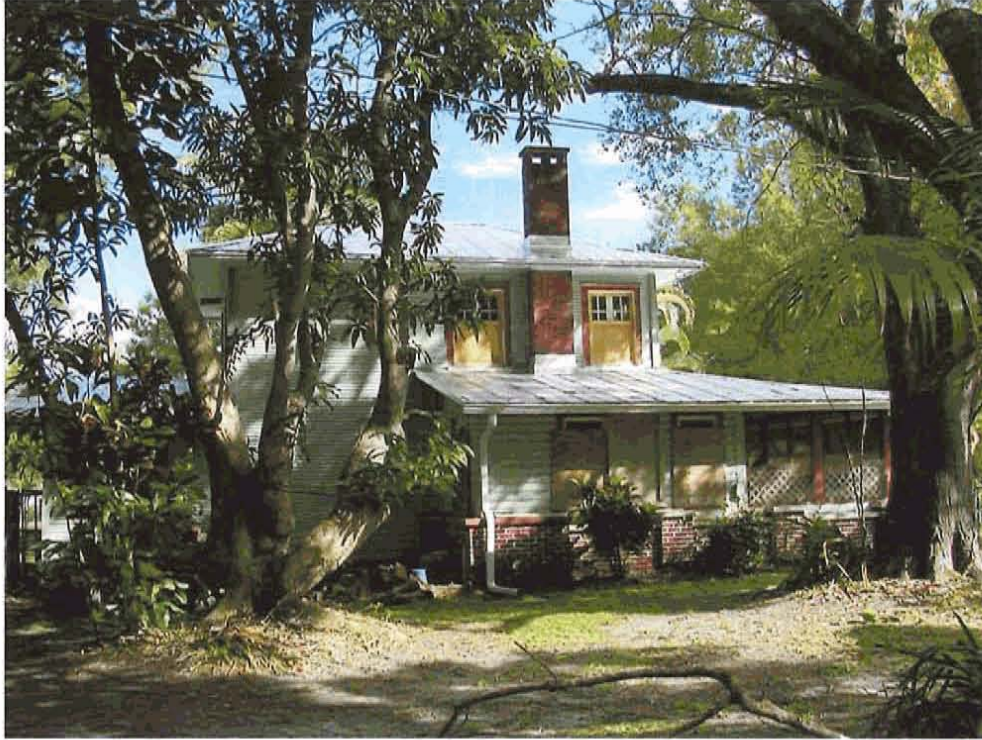
Right (south) elevation seen from Prospect Ave
