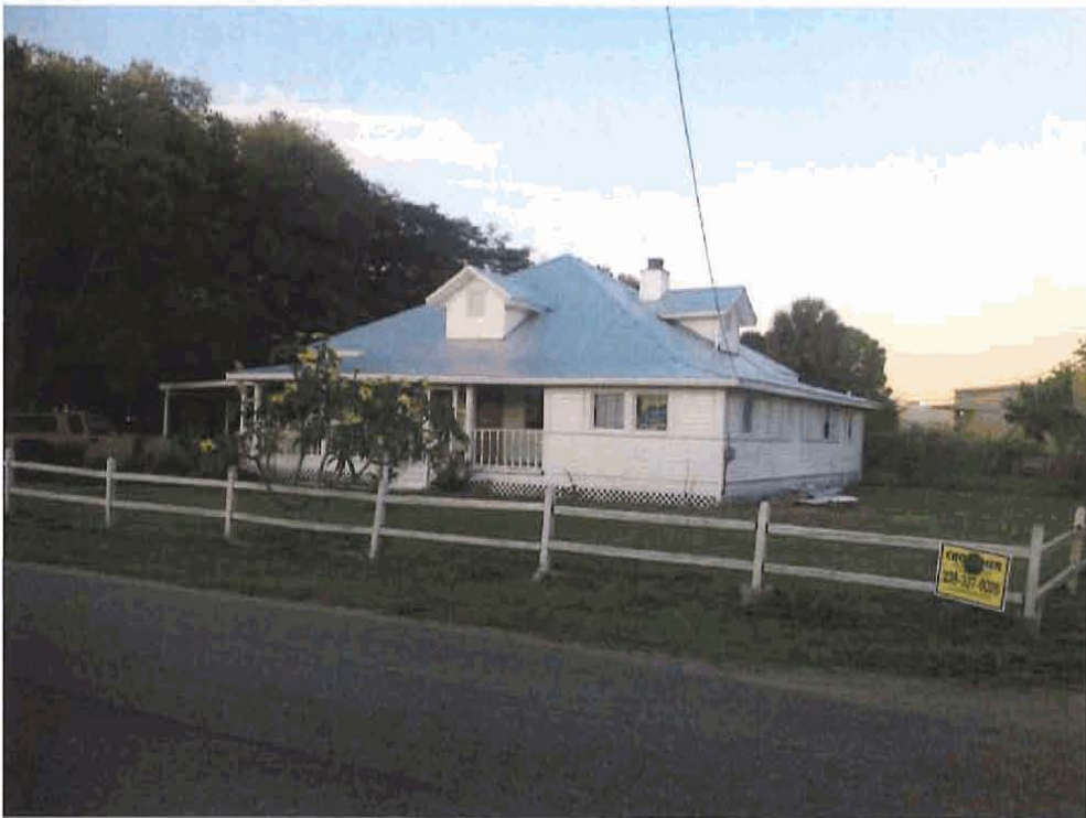
New roof completed
