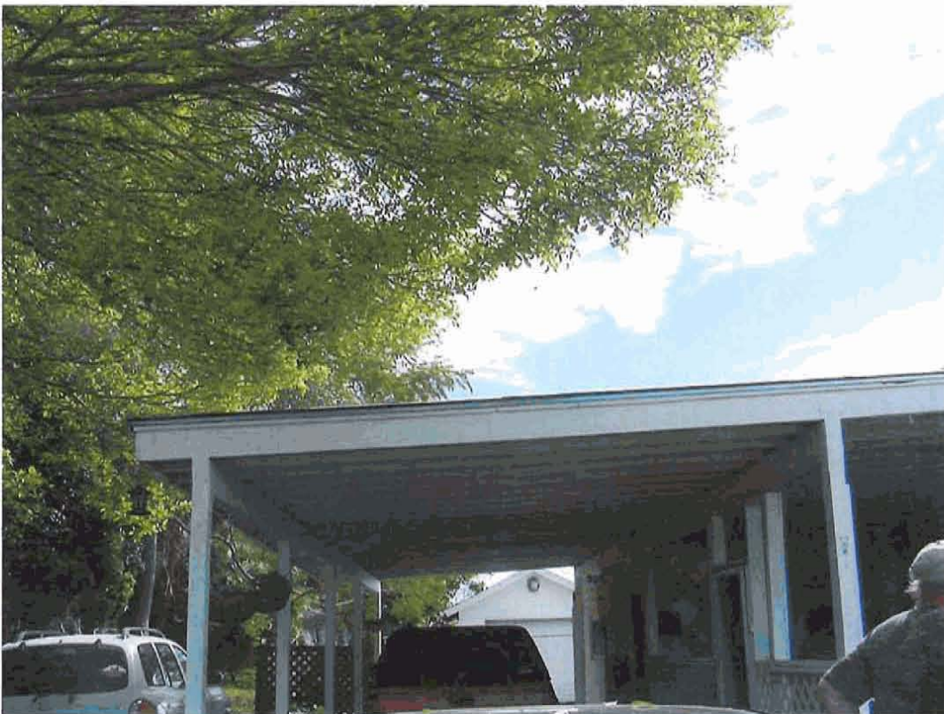
Carport on north side seen from the front
