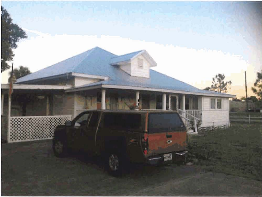
New roof completed
