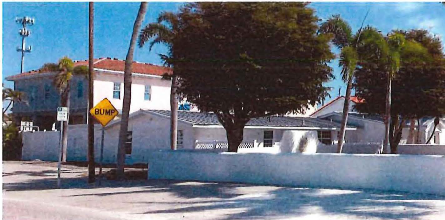
Figure 1. Existing building to be demolished
