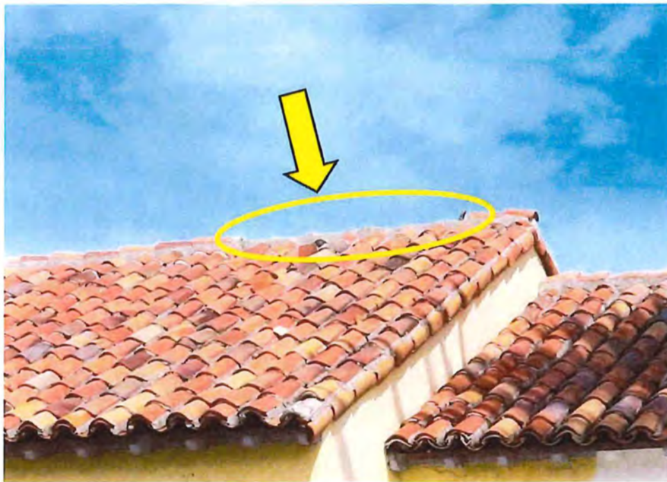
Figure 7. Multiple blown-off ridge tiles on building
