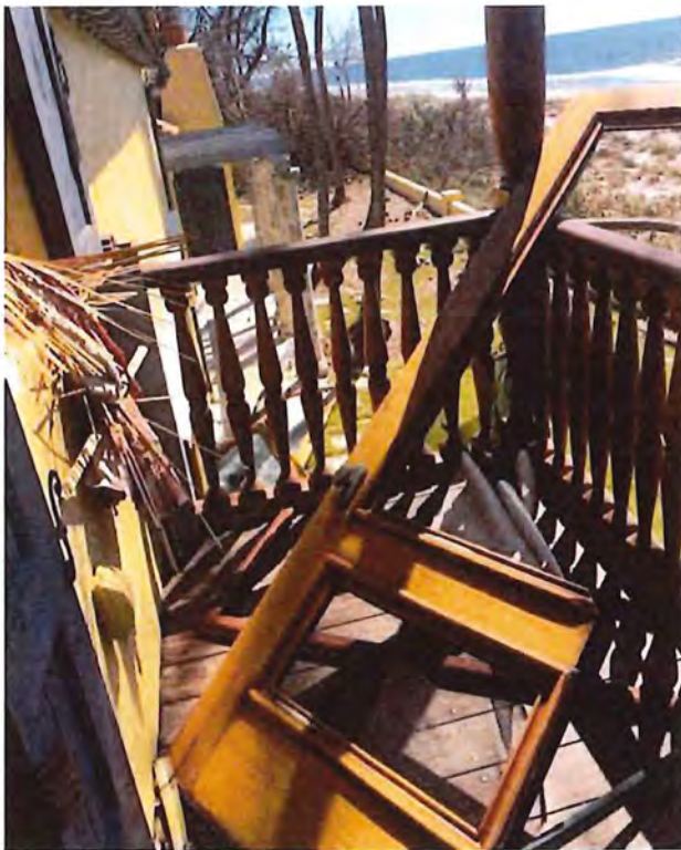
Figure 4. Typical post Hurricane Milton damage to fenestrations on second floor of main bldg.
