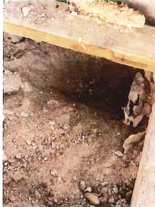
Close-up – Bearing depth approximately 8 inches
