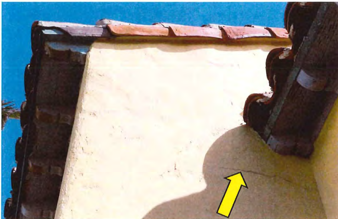
Figure 6. Cracking on stucco and masonry of exterior wall of main building
