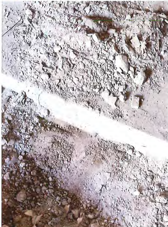
Interior slab edge – ~3 inches thick; no reinforcement observed
