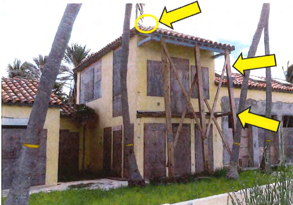
Figure 8. Temporary framing to support roof and exterior wall and missing ridge tiles on roof
