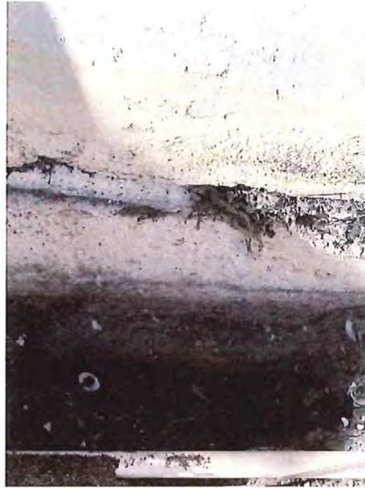
Close-up – Shallow stem wall (~8 inches below grade) with small footer
