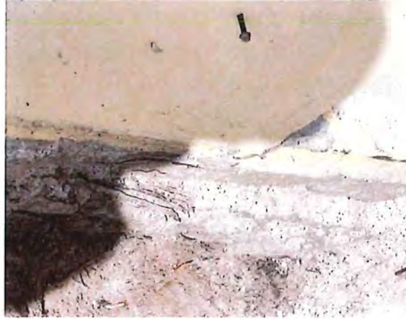
Close-up – Footer only ~6 inches below grade at B
