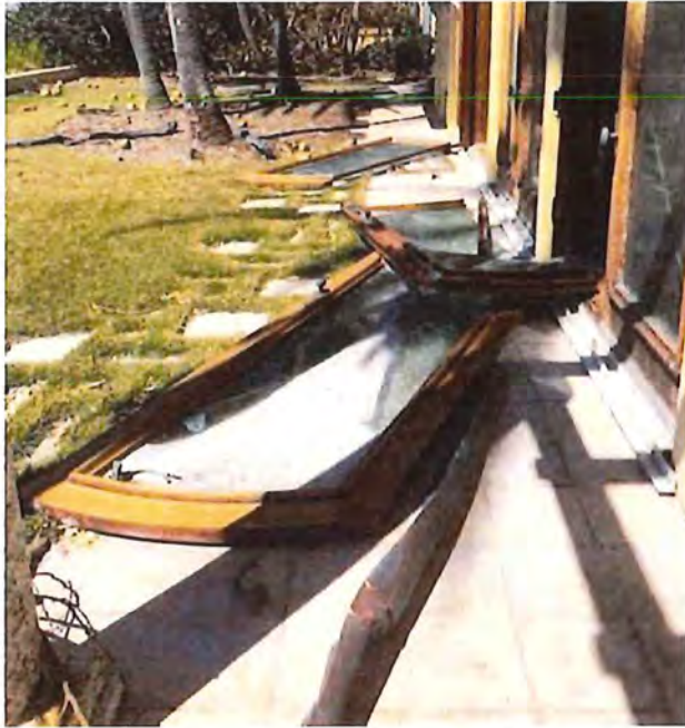
Figure 3. Typical post Hurricane Milton damage to fenestrations at the residence
