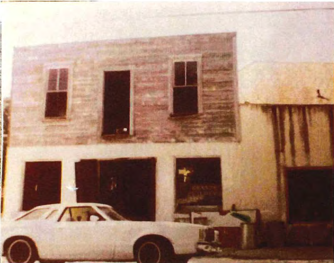
1980s photo of the building façade along 4 th St E of the building at 446 4 th St E. BG Note door opening on the second-floor level indicating an opening to a balcony or porch over the sidewalk. Source Braxton Bowen
