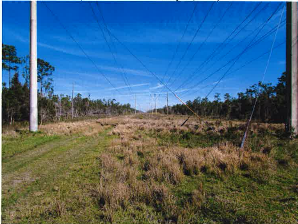
Transmission lines and easement (Photo Taken on February 17, 2017)
