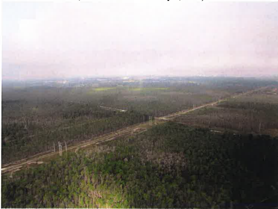
Aerial view of FP&L transmission lines (Photo Taken on February 9, 2017)
