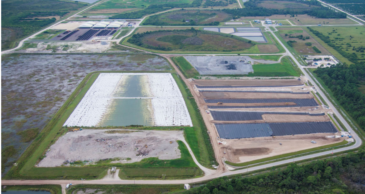
The Lee / Hendry Regional Landfill shown above includes an ash monofill, class I and class III landfill sites, leachate management and deep injection well, and the County's composting facility.
