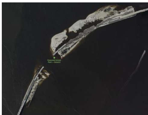
Figure 6: Image of a portion of the Sanibel Causeway showing the impact of Hurricane Ian; Source: National Oceanic and Atmospheric Administration Remote Sensing Division
