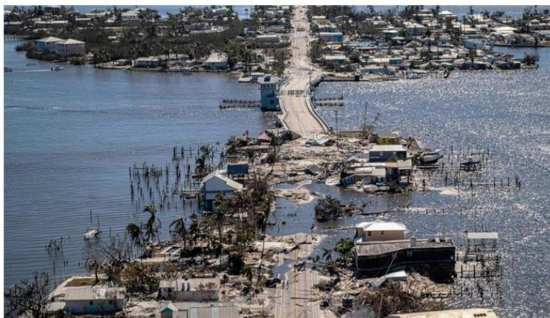
Figure 7: Image of Matlacha Bridge on September 30, 2023; Source: Agence France-Presse via Getty Images
