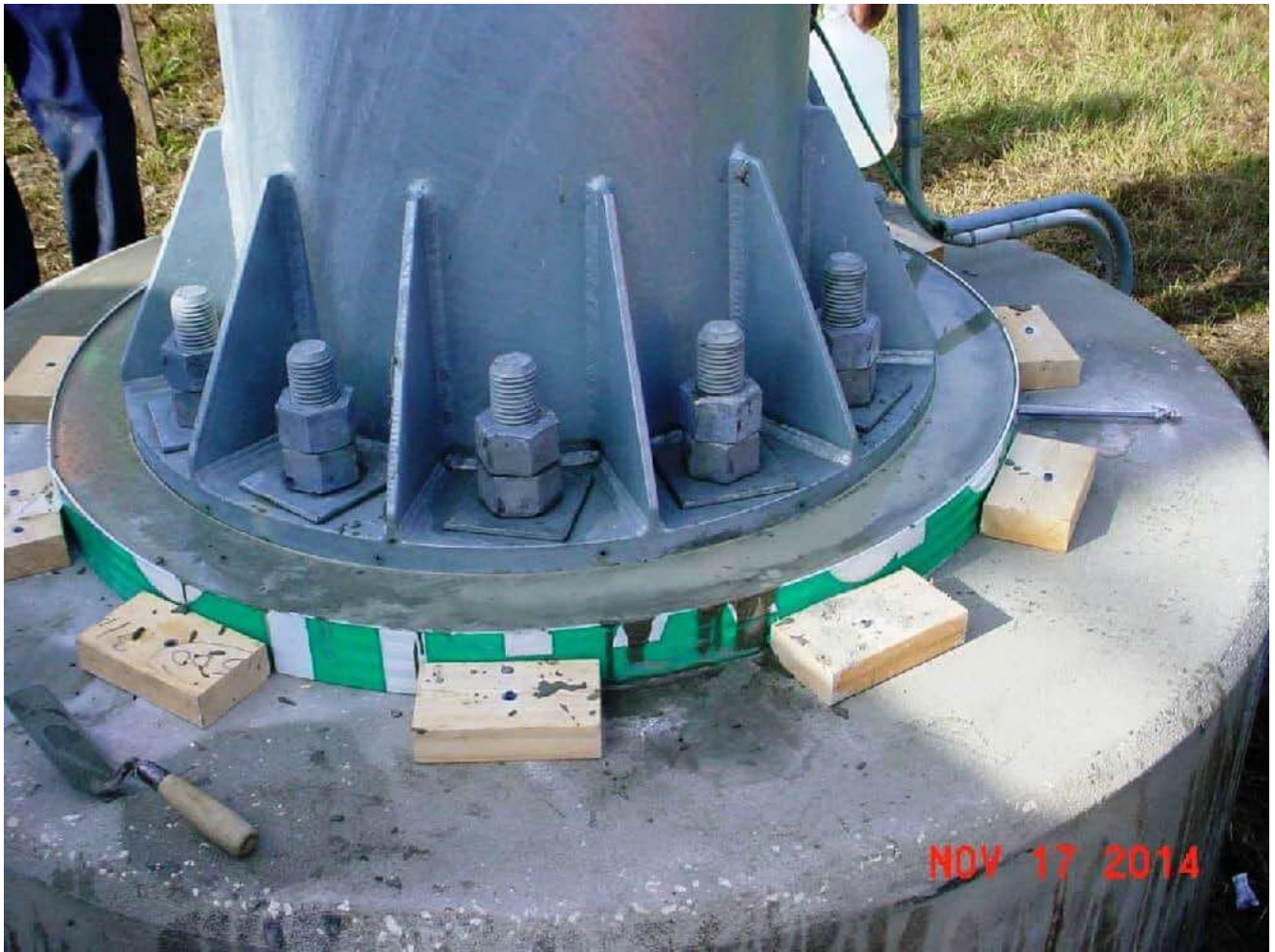
Typical grout filled form.
