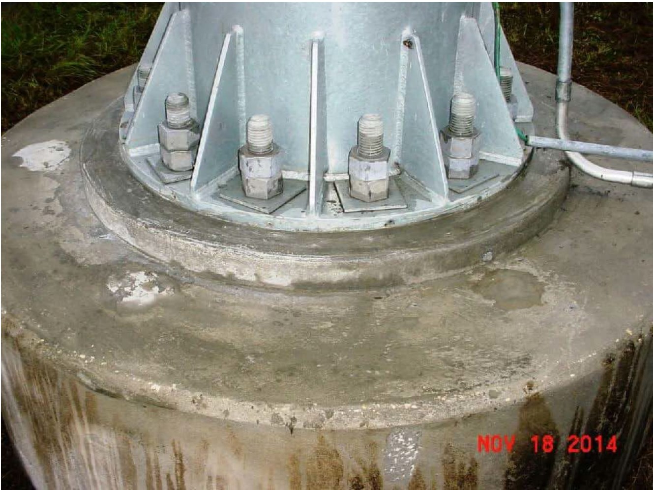
Typical completed structural grout pad.
