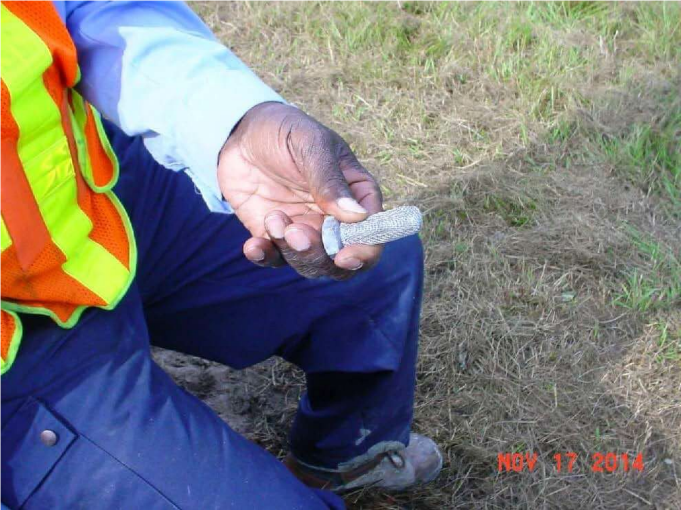
A piece of aluminum screen is then preformed around a bolt.
