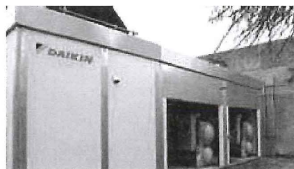
MCP with Dual Chillers Inside
