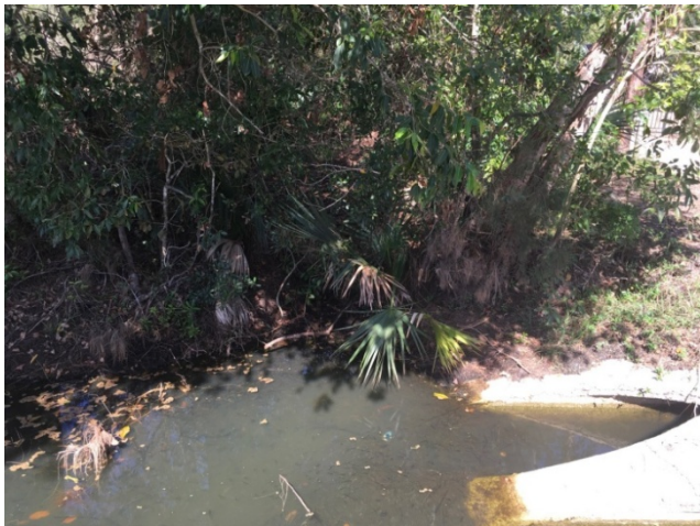
Receiving drainage ditch just east of Bayshore Creek access culverts *Data Point 1785 Lat: 26.7554 Long: -81.8181
