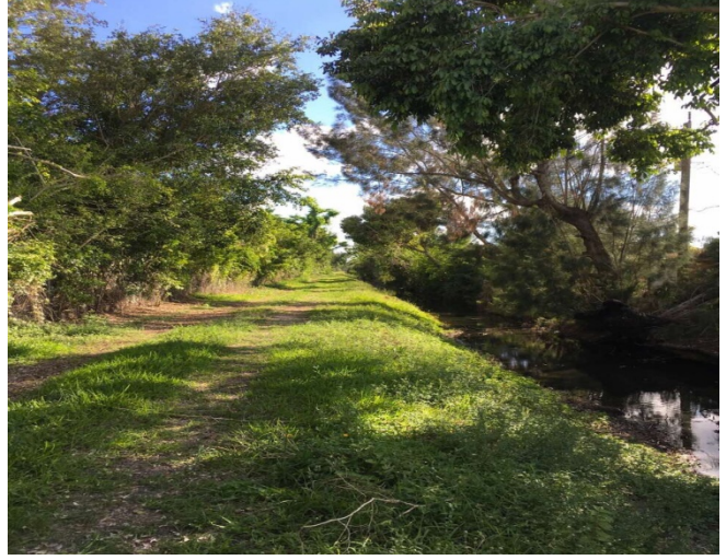
N/S Canal North of Trailwinds Dr., looking north *Data Point L35 Lat:26.57060536 Long:-81.86328131
