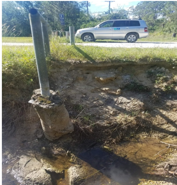
South of Nalle Grade Road culvert to Bayshore Creek looking north. Severe erosion caused at Bayshore Creek *Data Point 223 Lat: 26.7554 Long: -81.8181
