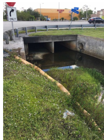
Brantley canal west of US 41.
