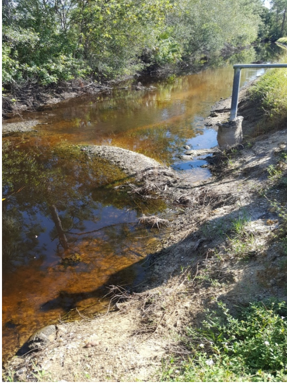
Sediment weir created by the erosion. *Data Point 223 Lat: 26.7554 Long: -81.8181
