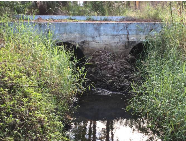
Debris & sediment blocking large diameter pipe @ 18681 Durrance Rd.
