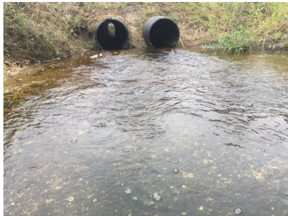
East side of Nalle Grade Road and Bowen Road.
