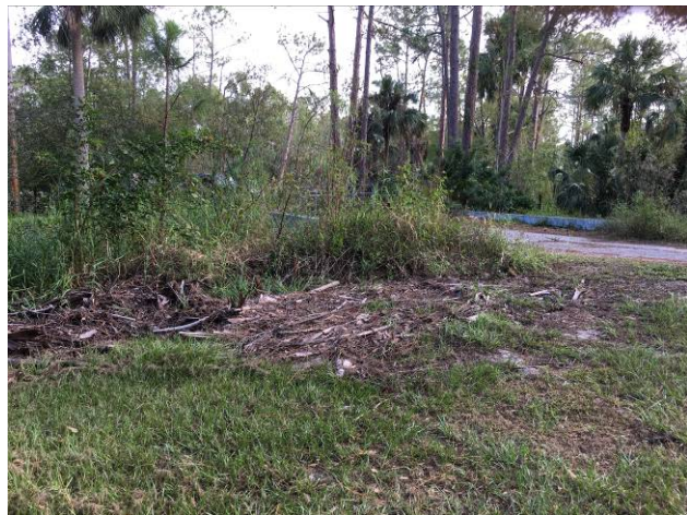
Debris indicating high water elevation
