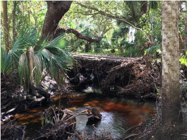
North side, north bridge, flood debris blocking about half section *Data Point 171 Lat: 26.718705 Long: 81.799410
