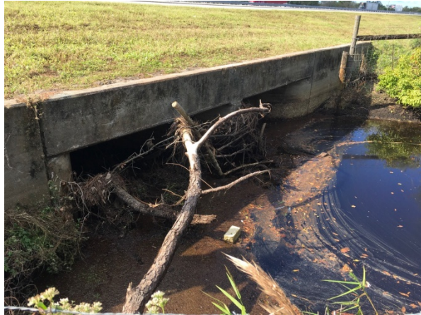
Northern culvert holding debris at I-75. *Data Point 1525 Lat: 26.72235 Long: -81.82409
