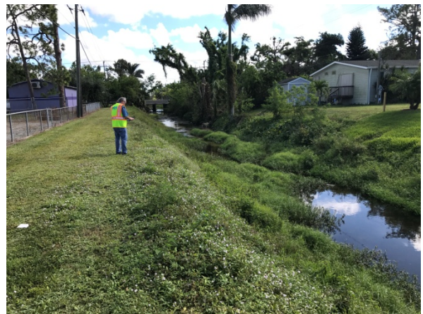
Looking east, L canal west of Danley Dr.
