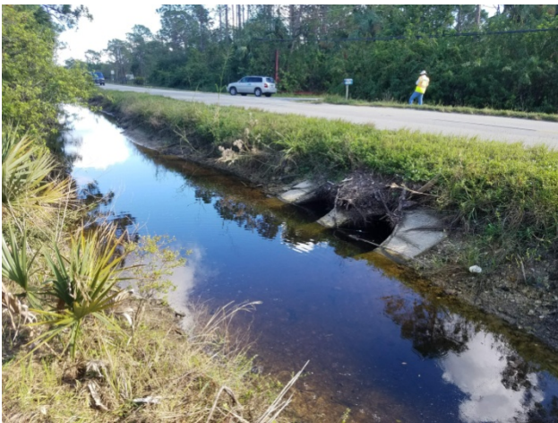
North side of Nalle Grade Road looking West. *Data Point 1586 Lat: 26.7555 Long: -81.8350
