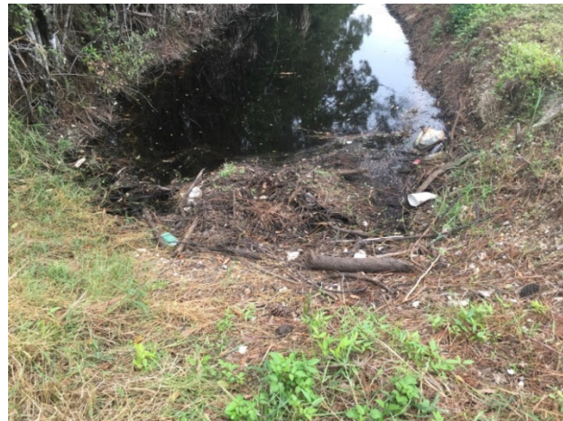
Debris build-up restricting flow on Nalle Grade Road. *Data Point 1014 Lat: 26.7555 Long: -81.8299
