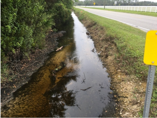
Looking East on East side of Nalle Grade Road and Williams Drive. *Data Point 849 Lat: 26.7555 Long: -81.8260
