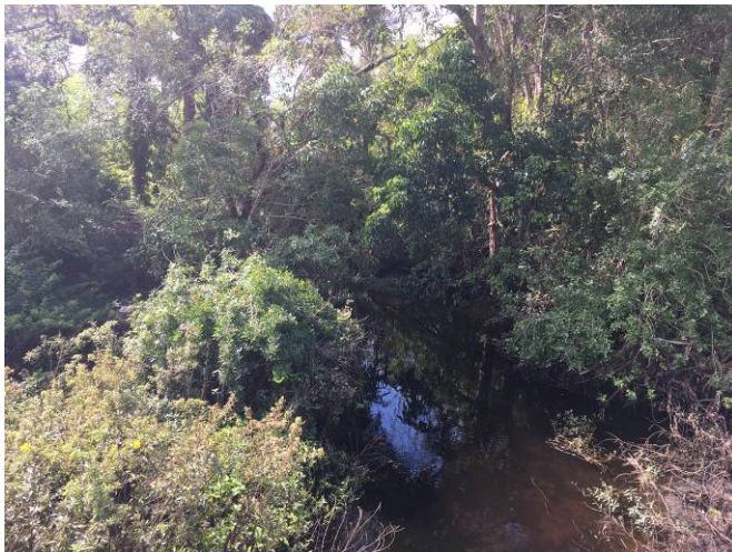
Looking south on bridge
