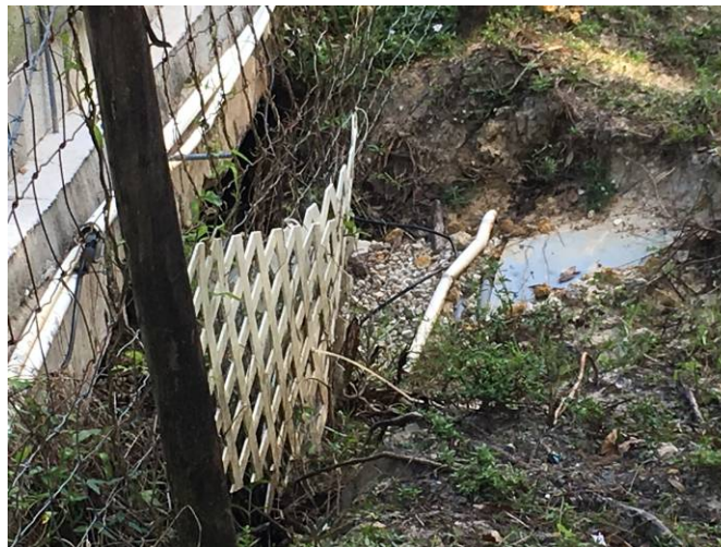
Water pushed thru under slab
