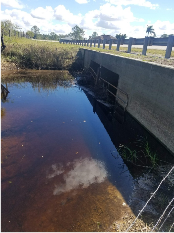
Gate with debris blocking flows at Pritchett Parkway. *Data Point 1499 Lat: 26.7638 Long: -81.8247
