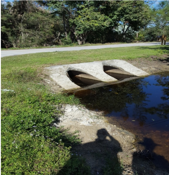
South of Nalle Grade Road culvert to Bayshore Creek looking north. Severe erosion caused at Bayshore Creek *Data Point 223 Lat: 26.7554 Long: -81.8181
