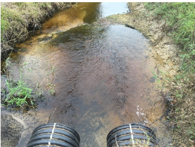
Sediment builds up creating a weir on East side of Nalle Grade Road and Bowen Road.
