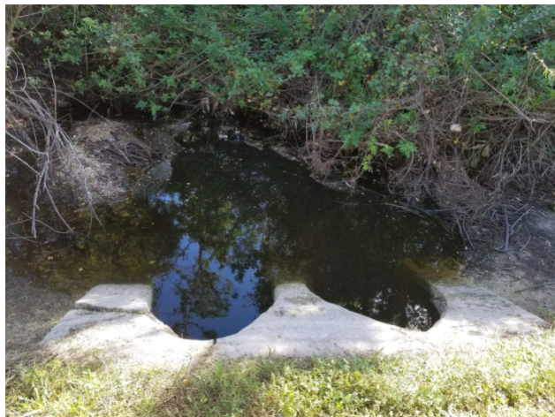
Drainage of Daughtrey's Creek East Branch south of Nalle Grade Rd *Data Point 1583 Lat: 26.7555 Long: -81.8350
