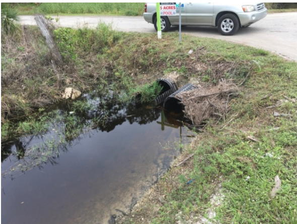
West side of Nalle Grade Road and Bowen Road.
