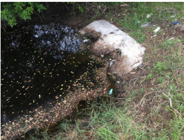
Moving East on Nalle Grade Road from Williams Dr. this is the West side of the next driveway culvert. *Data Point 1766 Lat: 26.7554 Long: -81.8251
