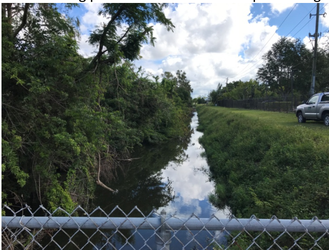
Along L canal at Danley Dr., looking east.
