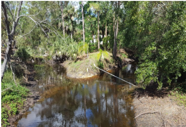
Looking North on Daughtrey's Creek Bridge. *Data Point 219 Lat: 26.7553 Long:-81.8514
