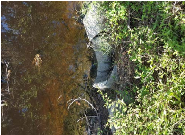
North/south culvert not accepting water due to high invert. *Data Point 1588 Lat:26.7554 Long: -81.8341
