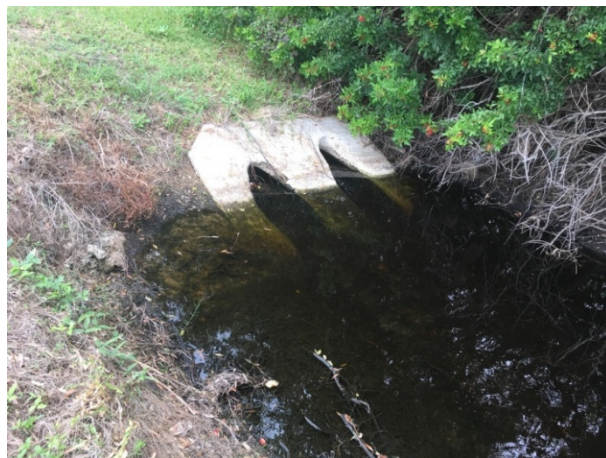
Moving East on Nalle Grade Rd from Williams Dr, this is the East side of the next driveway culvert. *Data Point 1766 Lat: 26.7554 Long: -81.8251
