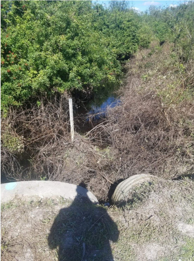
This picture is looking north on the north side of Henderson grade showing the overgrown vegetation. *Data Point 216 Lat: 26.7426 Long: -81.8186
