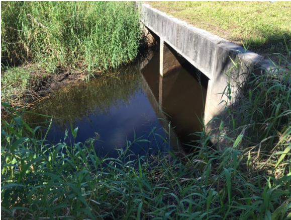
Southern culvert outlet showing 50% blockage due to overgrowth and sediment build up at I-75. *Data Point 1526 Lat: 26.72235 Long: -81.82409
