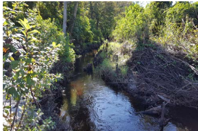
South culvert of Bayshore Road looking downstream. *Data Point 1495 Lat: 26.71478 Long: -81.8217
