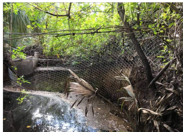
Looking south water gap fence debris behind
