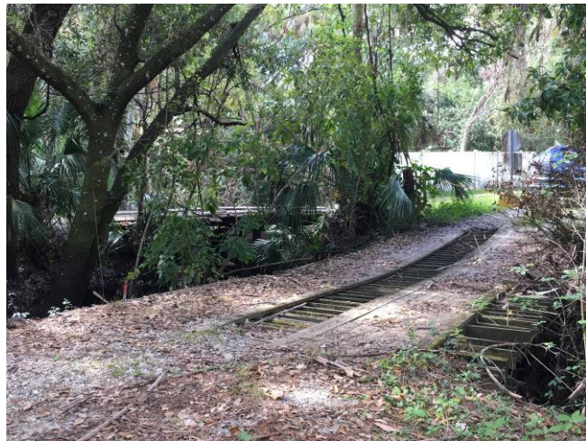
2 private bridges looking south *Data Point 171 Lat: 26.718705 Long: 81.799410
