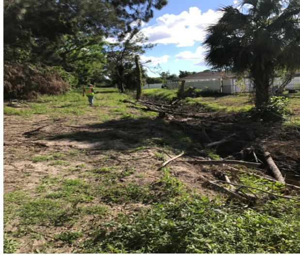
Debris in N/S canal south of Trailwinds Dr. *Data Point L34 Lat:26.5678 Long:-81.86329
