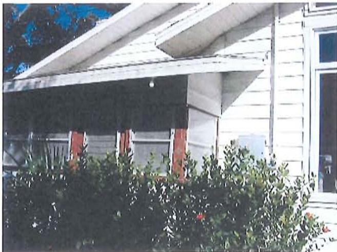
Front (North) elevation by N. River Rd
