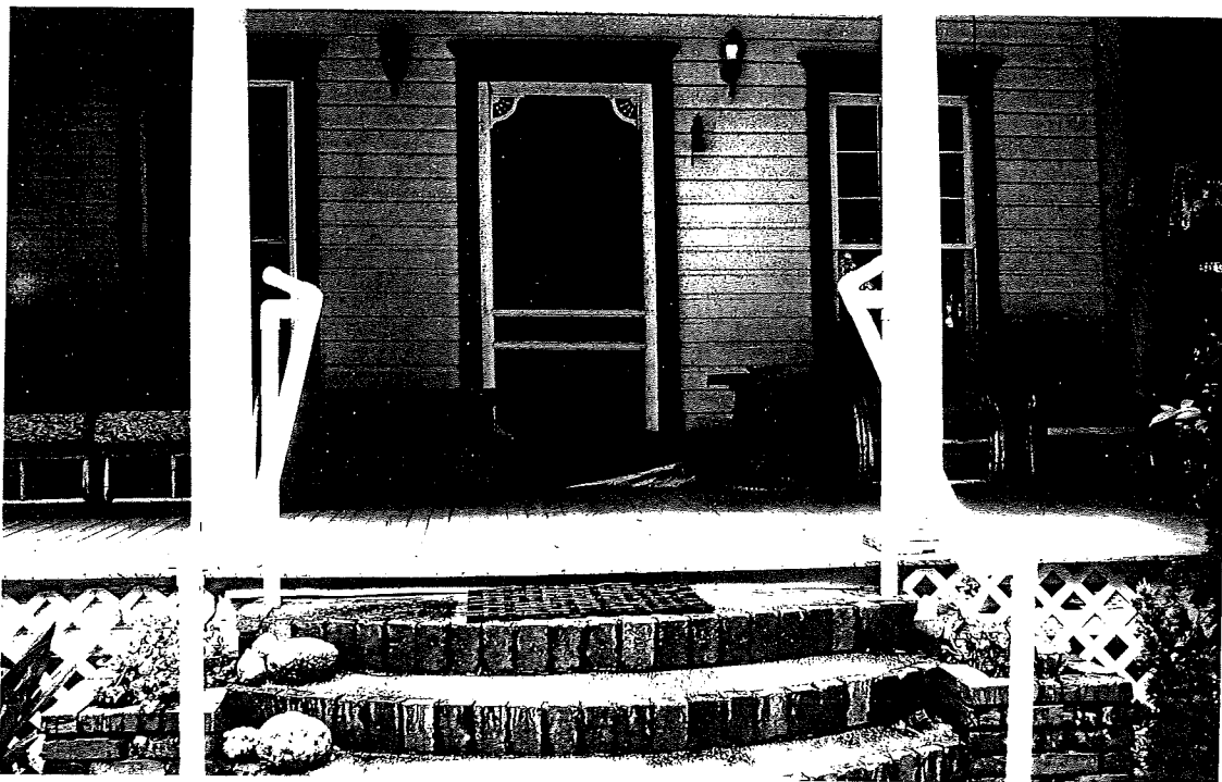
Detail of the south elevation's porch
