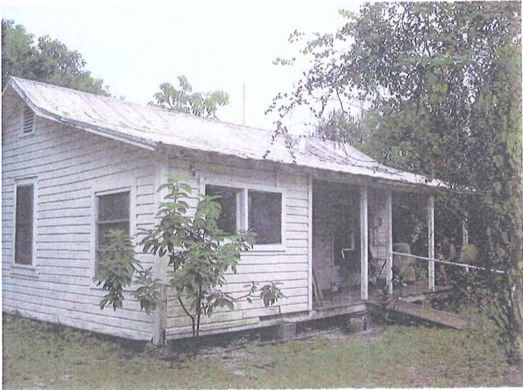
Front (north) and partial east side
