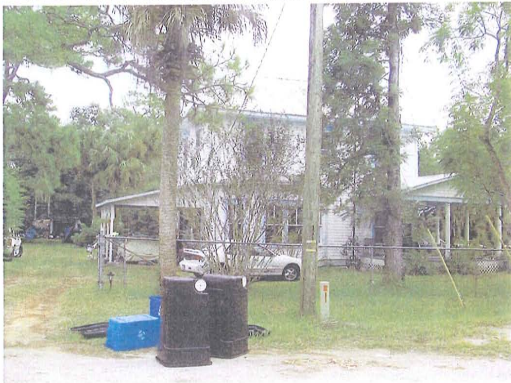
Street front - west
