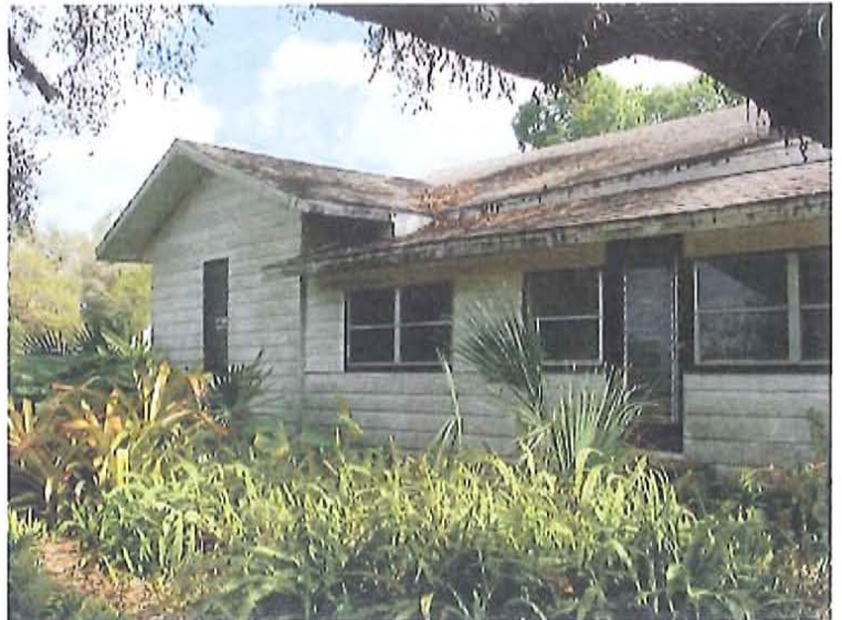
Side (West) facing Telegraph Creek
