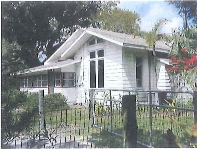
Front (North) elevation by N. River Rd
