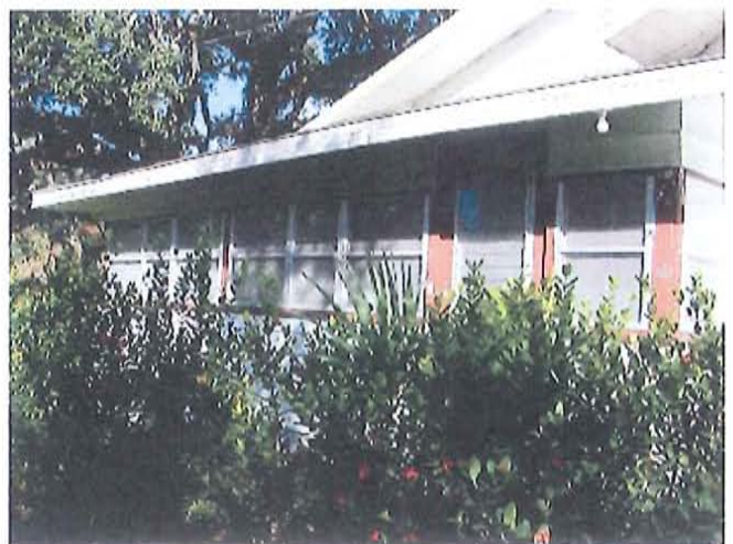
Front (North) elevation by N. River Rd
