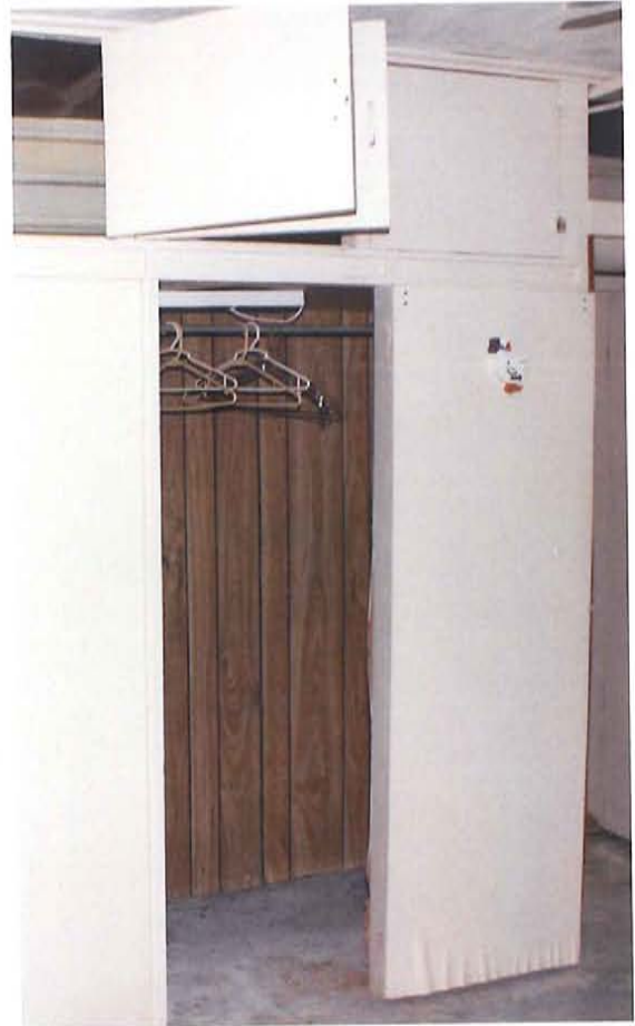
Above left: north side of cottage. Above right: Bedroom closet, showing original siding behind upper cupboards and water damage at floor level. Below: east side of property with cistern.
