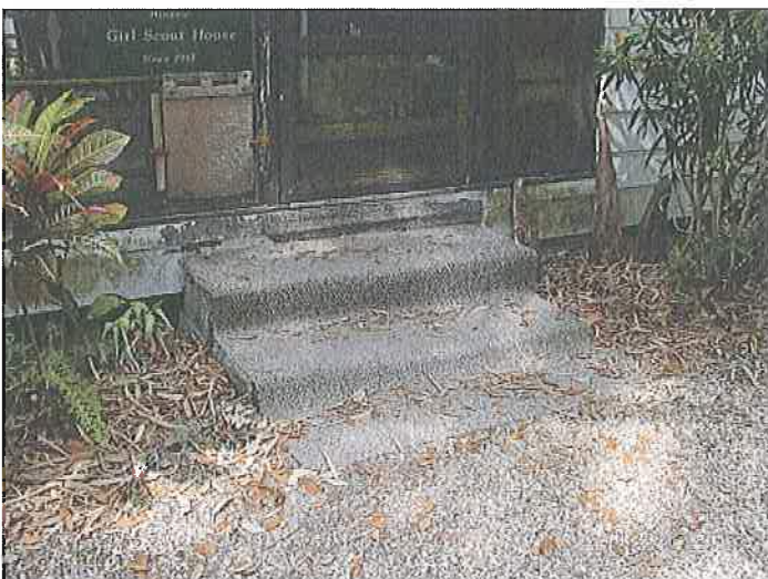
Porch stairs to be removed
