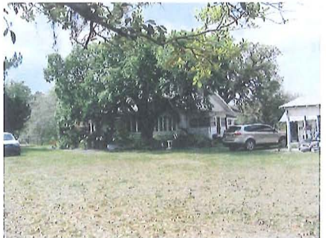
Rear South and partial of side East
