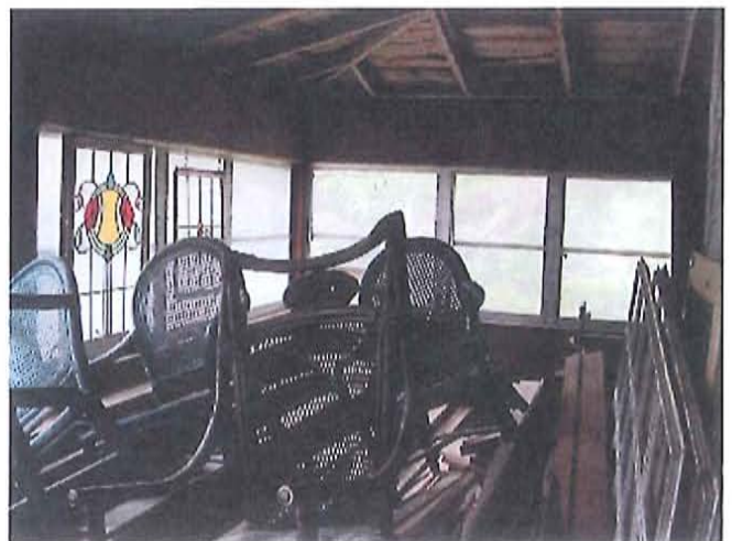
Front wrap around porch to be rehabbed
