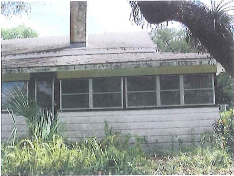
Side (West) facing Telegraph Creek
