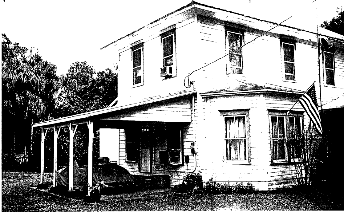
north and west elevations
