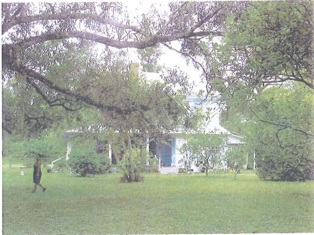
East or rear of the existing historic building
