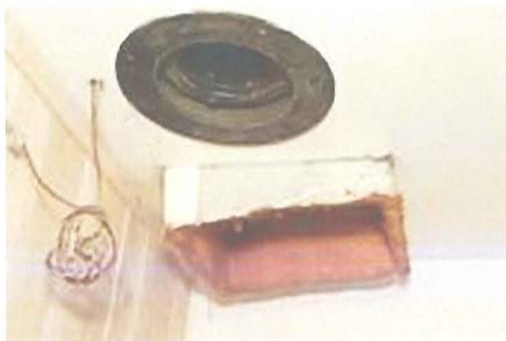
Utility Room Ceiling (Room for Fire Wall Construction)
