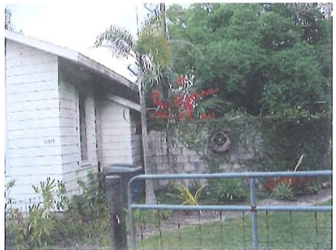
Front (North) elevation by N. River Rd
