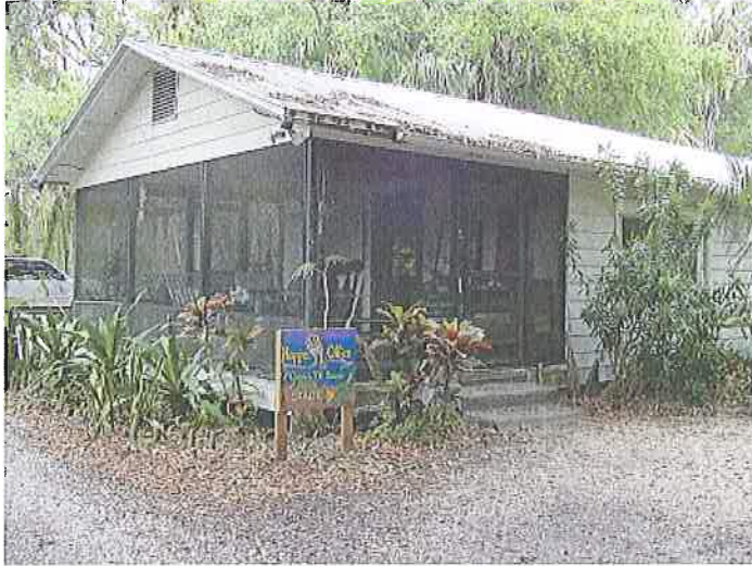
Northwest entrance porch
