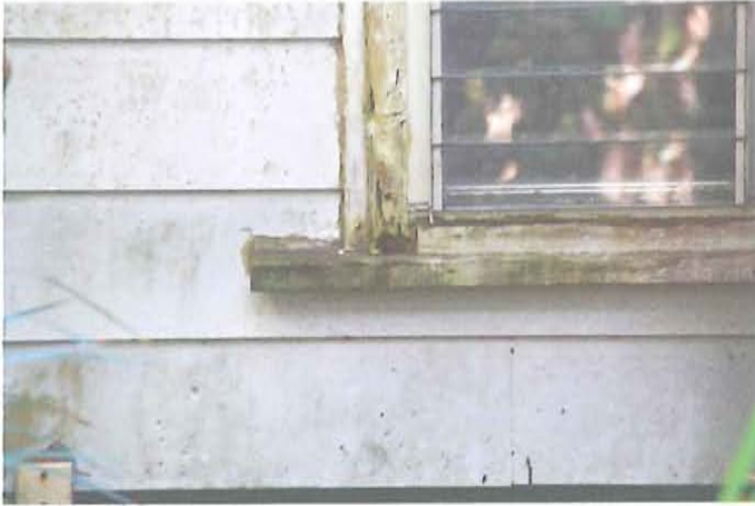
Rotting Window Sills
