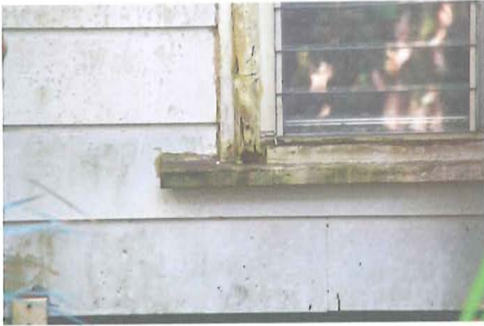
Rotting Window Sills
