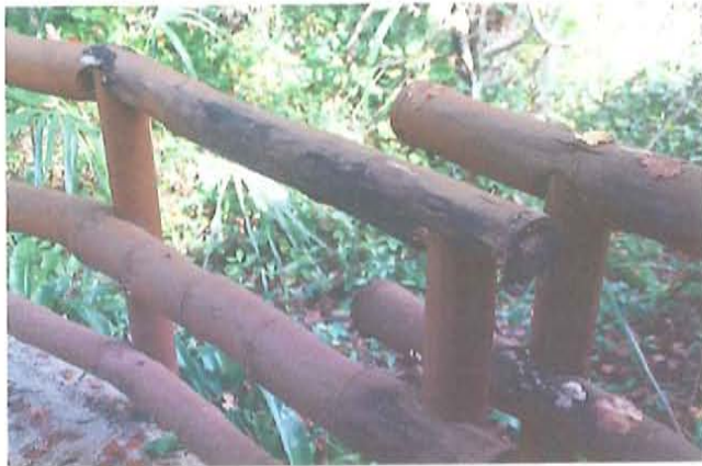
Handrails on Handicapped Ramp
