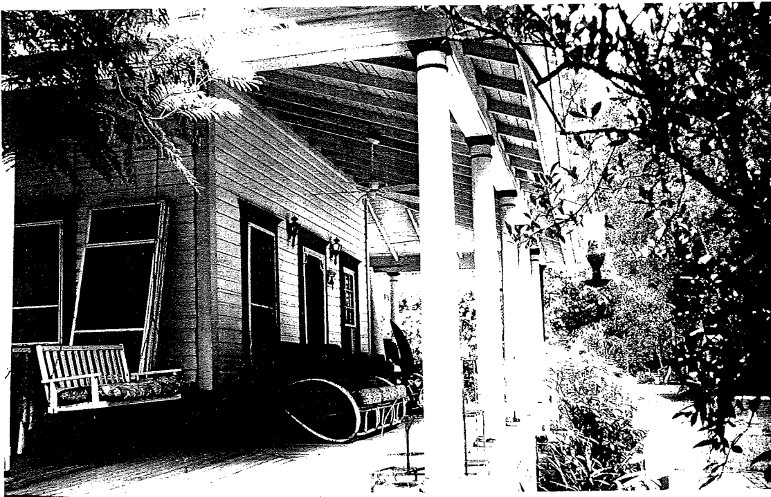
Detail of the south elevation's porch
