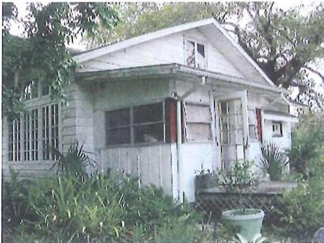
Rear South and partial of side East
