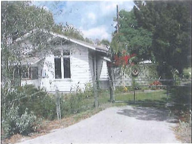
Side East and partial front North – note decorative fence wall
