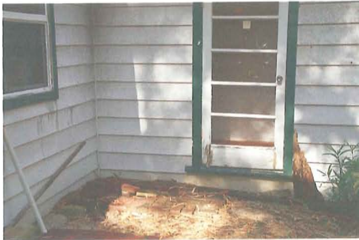
Rear Yard Exit Door and Proposed Space for Deck
