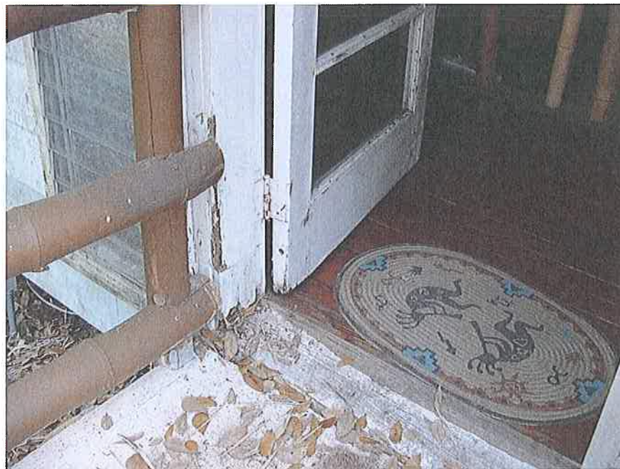
Door surrounds and approach (North)
