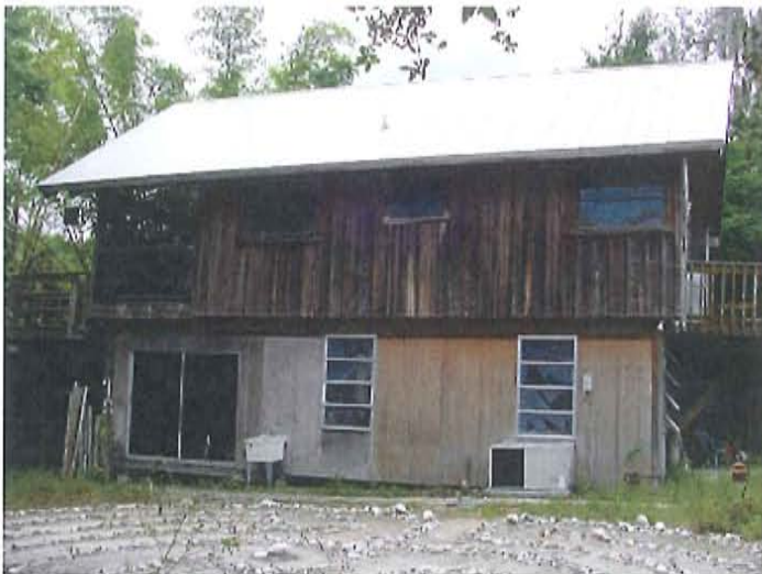
“Ellen’s River House” - Single family house across and north of the Estero River
