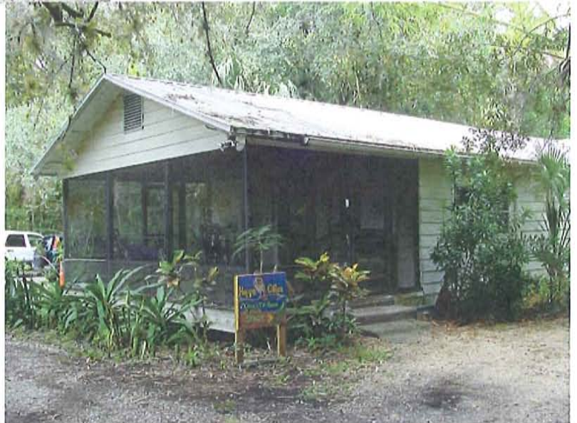
North wing – South side and front screened porch incised under the main roof
