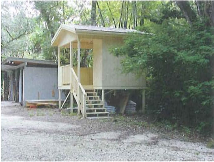
Composting toilet facility
