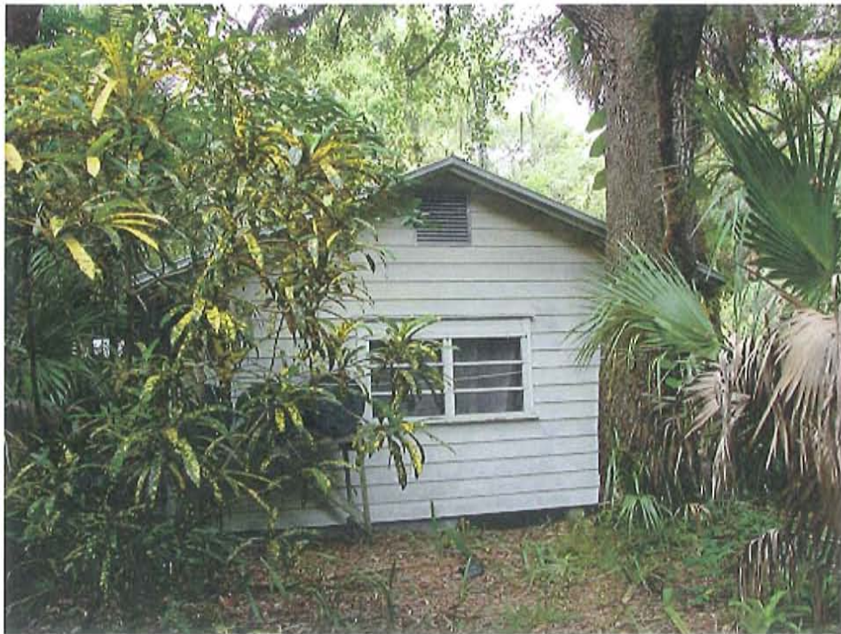
South wing – gable end
