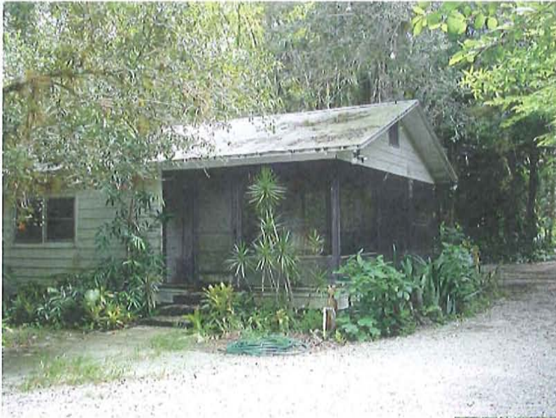
North wing – front (west) screened porch incised under the main roof
