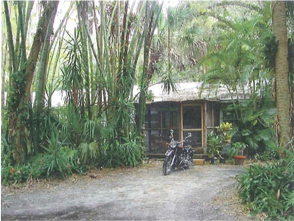
South wing: west side elevation with flat roofed porch (caretaker's residence)
