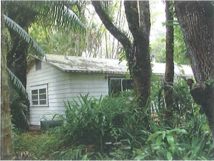
South wing: south gable end and east elevation
