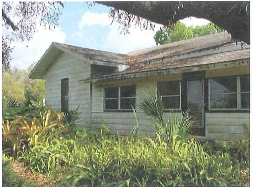
Side (West) facing Telegraph Creek
