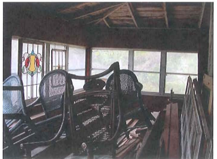
Front wrap around porch to be rehabbed
