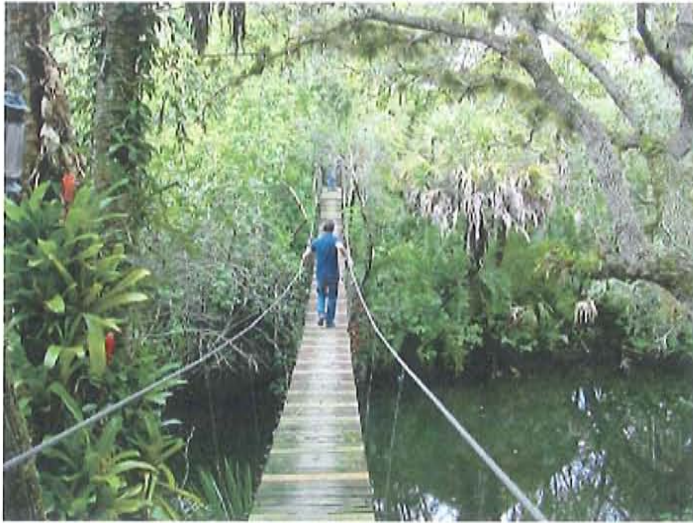
Swinging pedestrian bridge across Estero River
