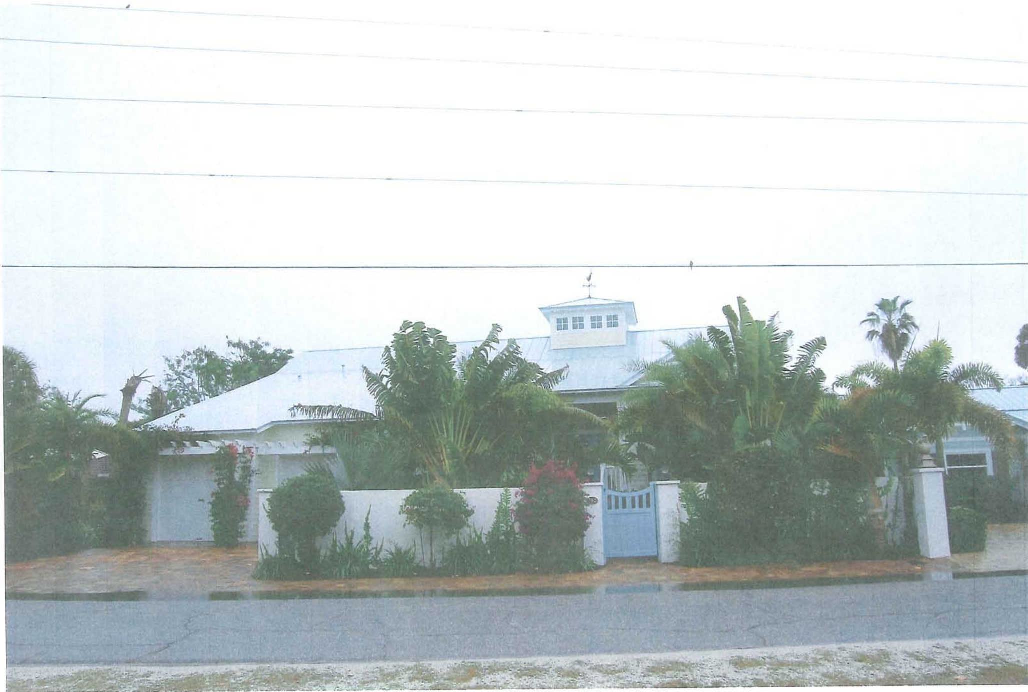
Photo 2 - 760 East Railroad Ave.
