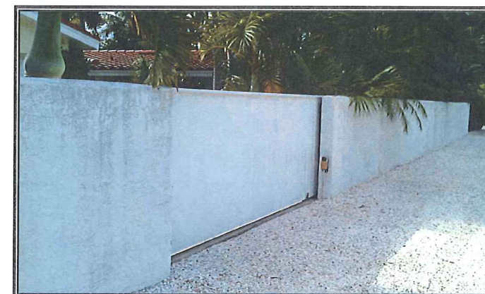
1060 EAST RAILROAD AVE. (SOUTH NEIGHBOR)
