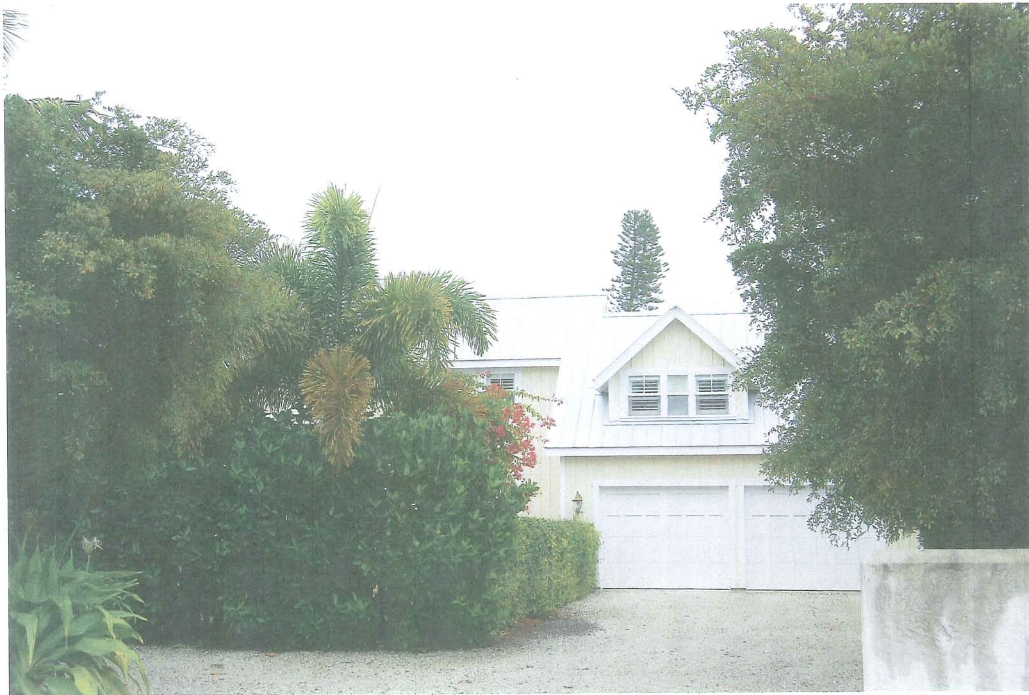
Photo 3 - 870 East Railroad Ave.
