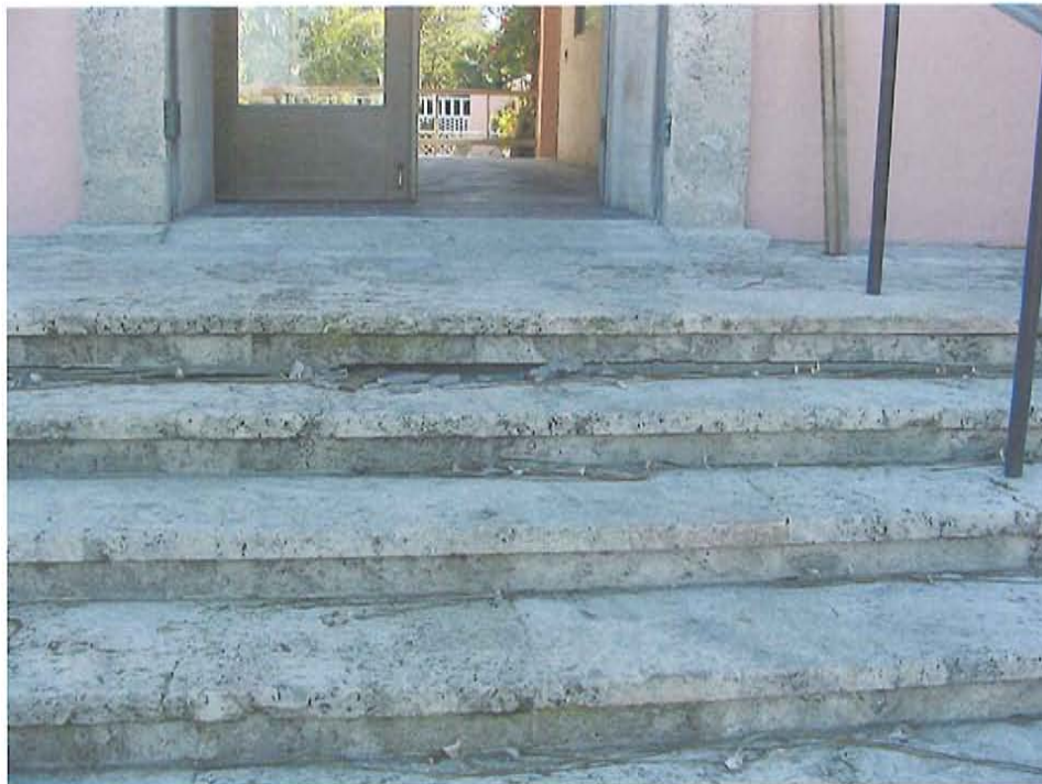
As steps have sunk a gap appeared between the top step and the landing. Note: over the years the gap was patched with cement
