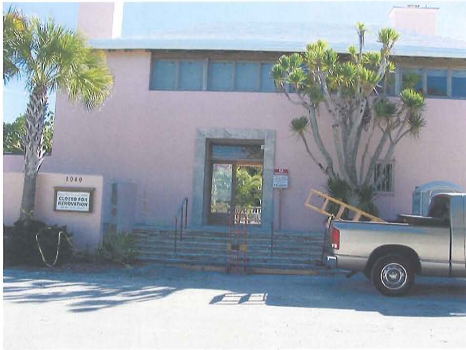
Front façade of the Fust Library – front steps to be replaced
