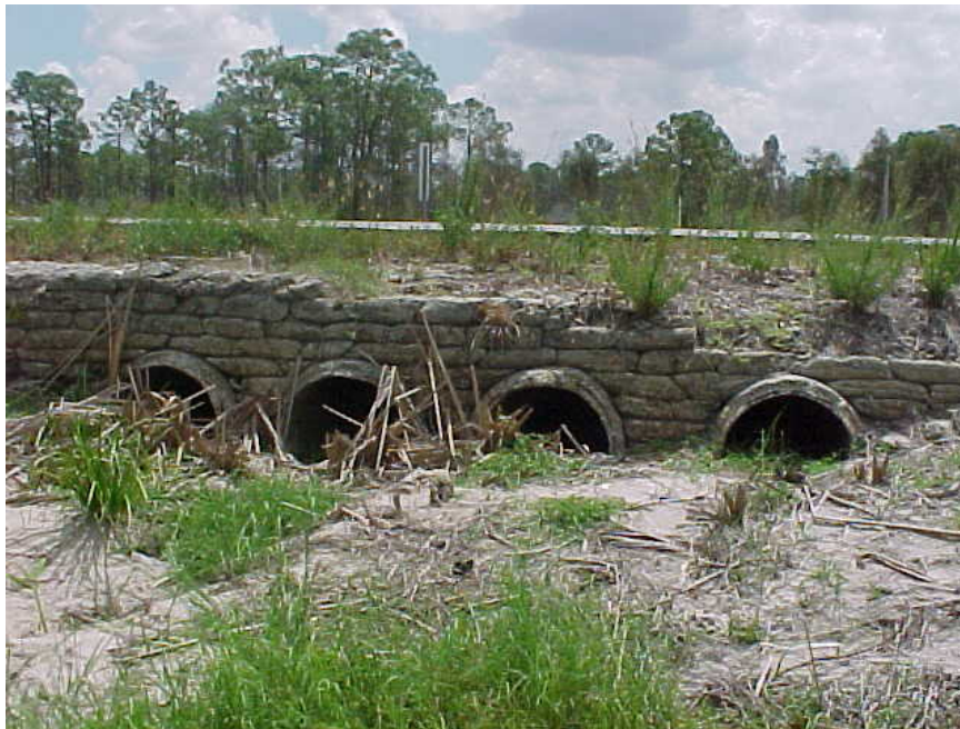
Culvert #4 – Downstream Side Headwall
