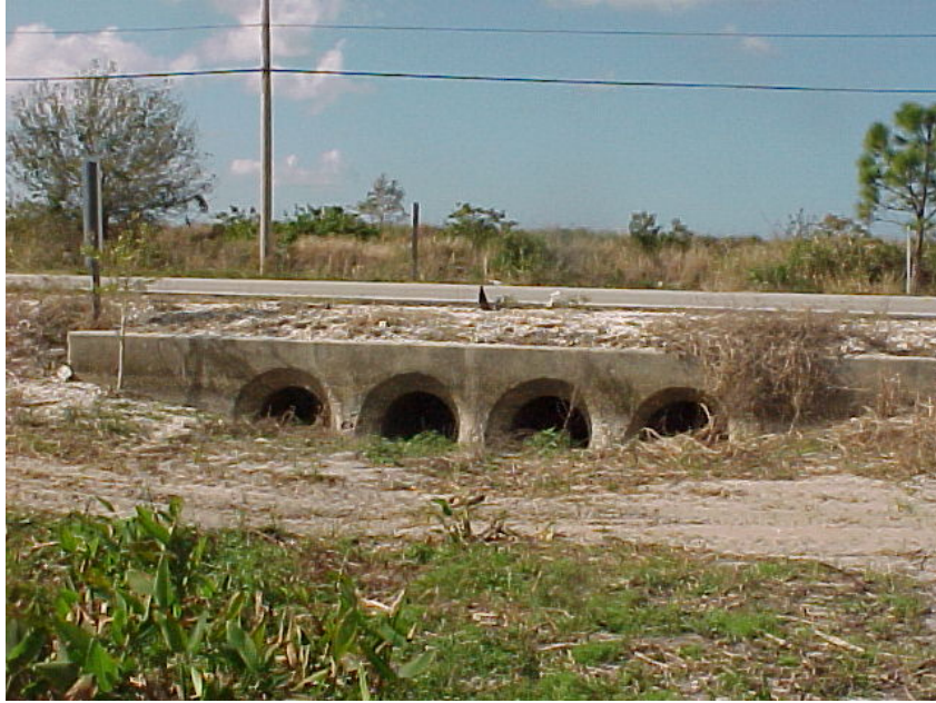
Culvert #4 – Greenwell Branch North at Burnt Store Road
