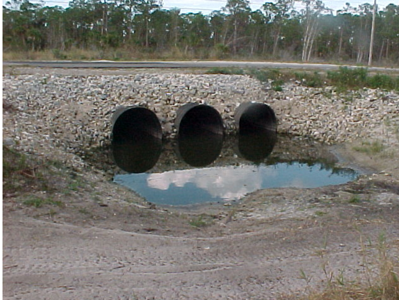
Culvert #3 – Durden Creek Main at Burnt Store Road
