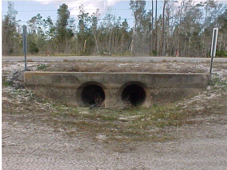
Culvert #2 – Durden Creek North Branch at Burnt Store Road
