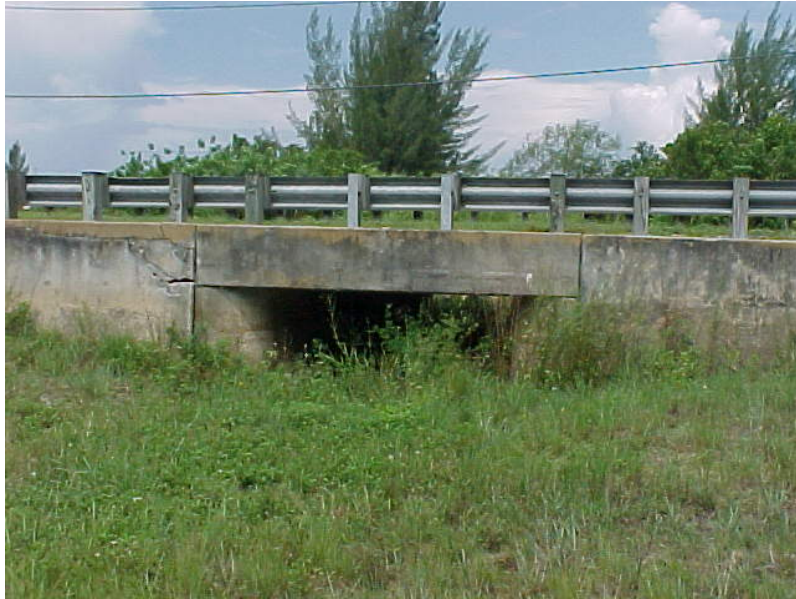
Culvert #9 South of Gator Slough Bridge at Burnt Store Road
