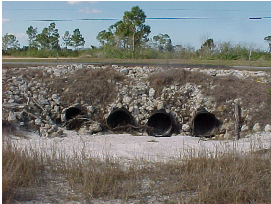
Culvert #5 – Greenwell Branch Main at Burnt Store Road
