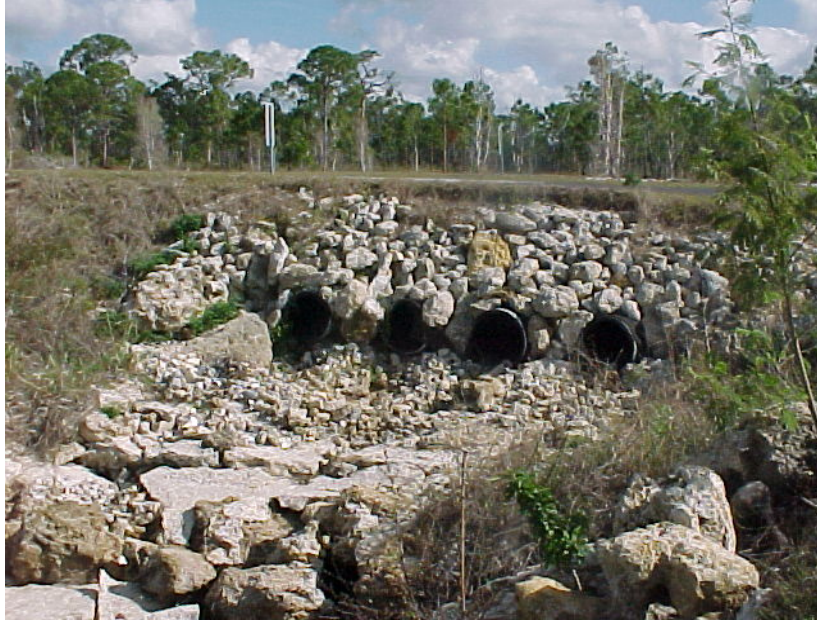
Culvert #5 – Downstream Face
