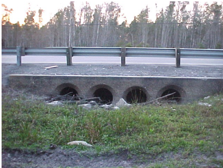
Culvert #6 at Burnt Store Road
