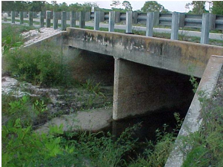
Culvert #1 – Yucca Pen Creek at Burnt Store Road
