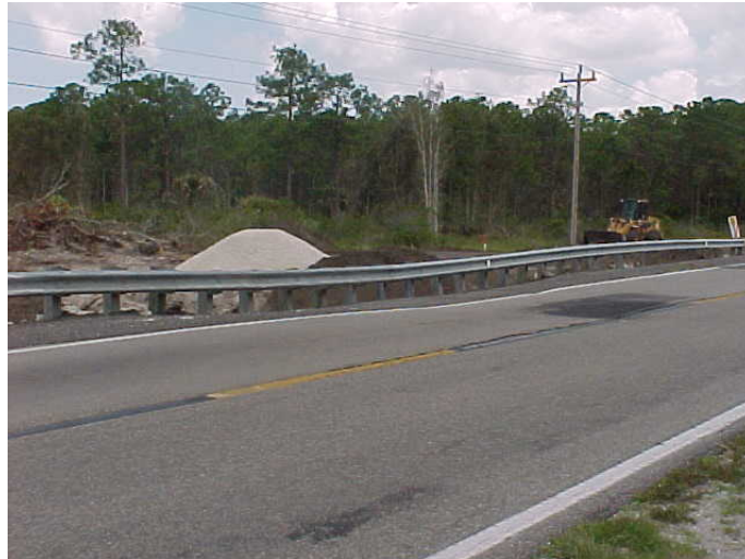
Failure of Durden Creek Main Culvert at Burnt Store Road during the June 2003 Event
