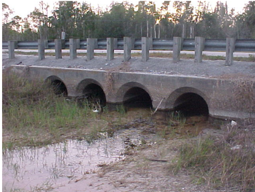
Culvert #8 at Burnt Store Road
