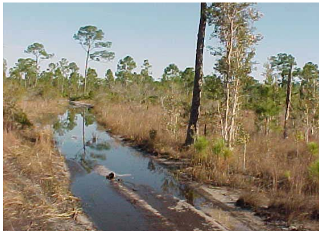
A Typical Shallow Flow Path/Vehicular Access Way Acting as a “Conveyance Channel”
