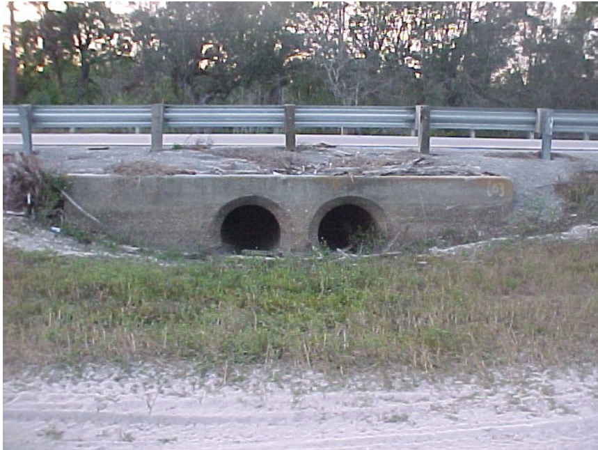
Culvert #7 at Burnt Store Road
