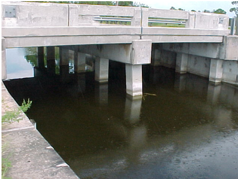
Culvert #10 (Bridge) at Burnt Store Road
