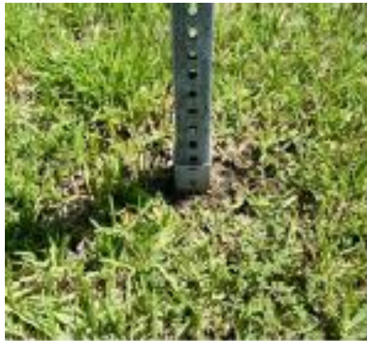
Typical Sleeve with Post construction
