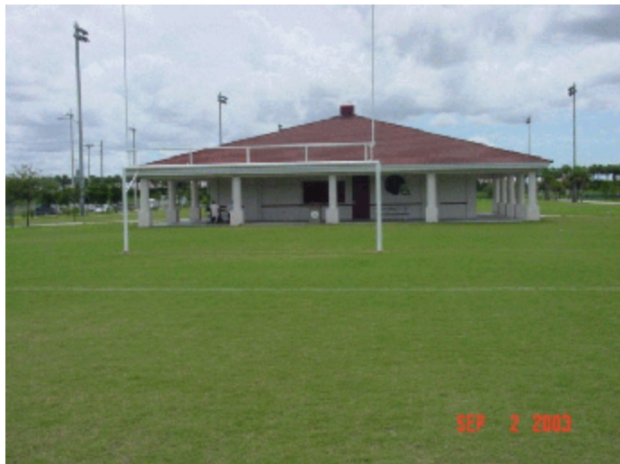
Multi-purpose fields and concession stand at Estero High School Park.
