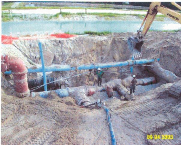
Installation of piping at the Reverse Osmosis plant for Bonita Springs Utilities.
