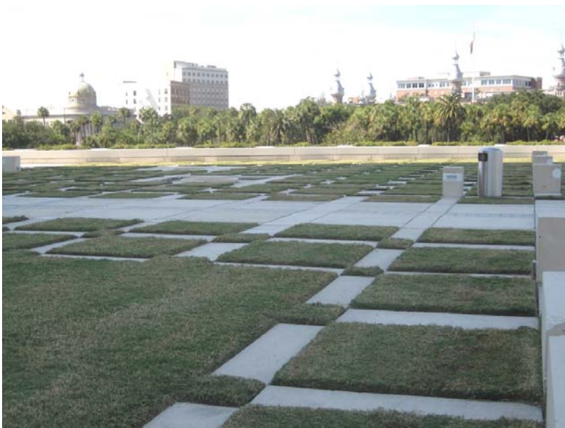
Green roofs can be an effective way to capture and treat stormwater while reducing energy consumption related to heating and cooling.
