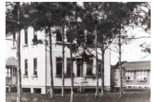
Edgewood School, built in 1911, destroyed by fire in the early 1980s (Board & Bartlett)
