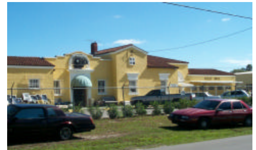
Reilly Bros., the former terminal for the Seaboard Airline Railroad, built in 1927
