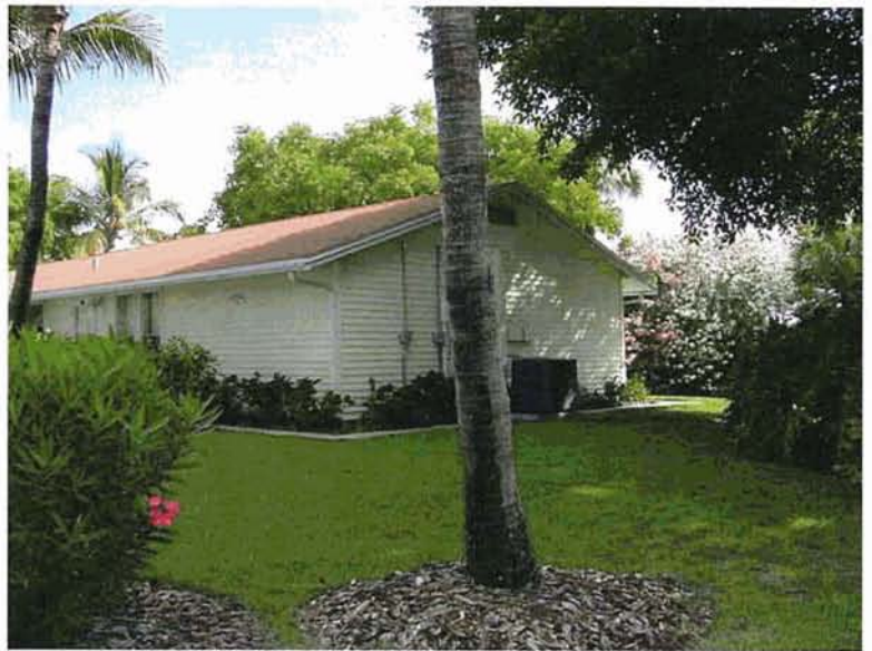
Front West and side South elevation along Palm Ave.
