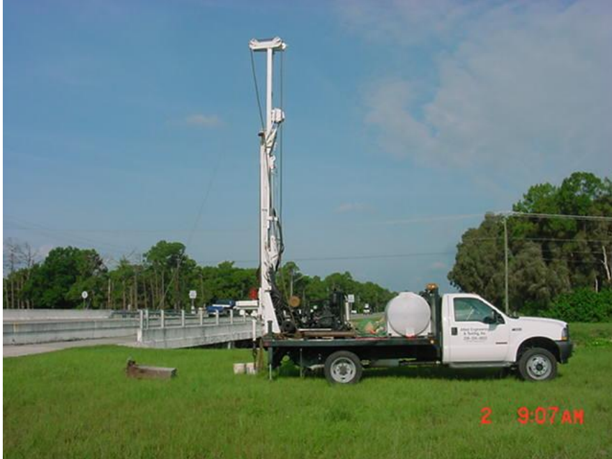
June 2, 2003 Soil borings north of Daniels Parkway.
