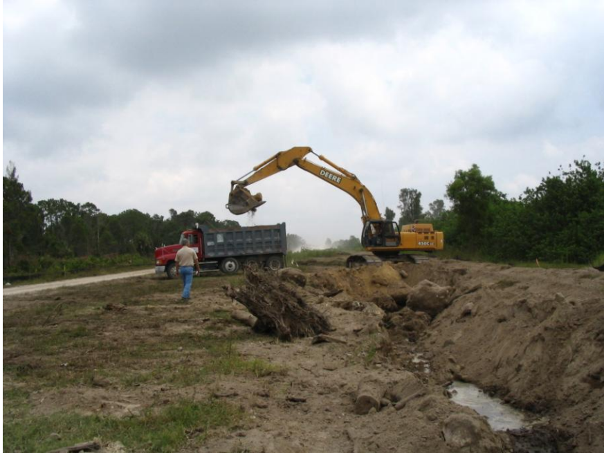
March 28, 2005 Excavation of the filter marsh cells and hauling dirt.
