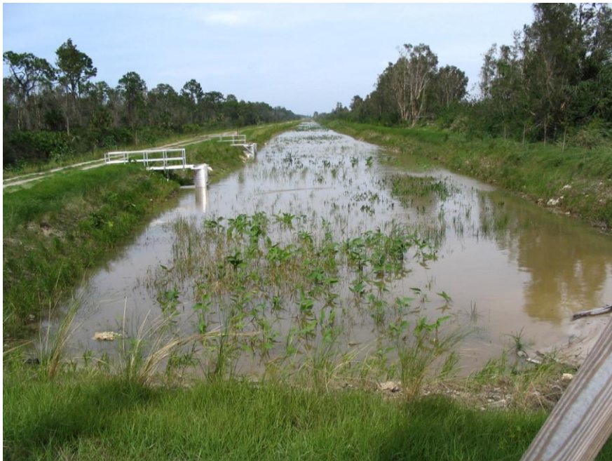
October 24, 2005 Cell No. 4 immediately after construction is complete. Looking north.
