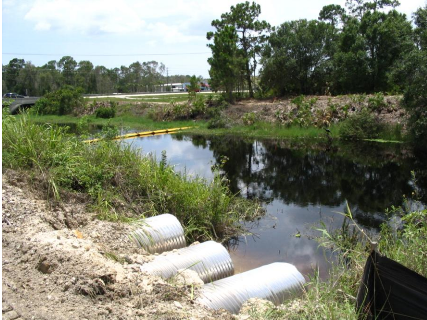
June 6, 2005 Filter Marsh discharge back into canal through 3 pipes from Cell No.4. Looking southwest.
