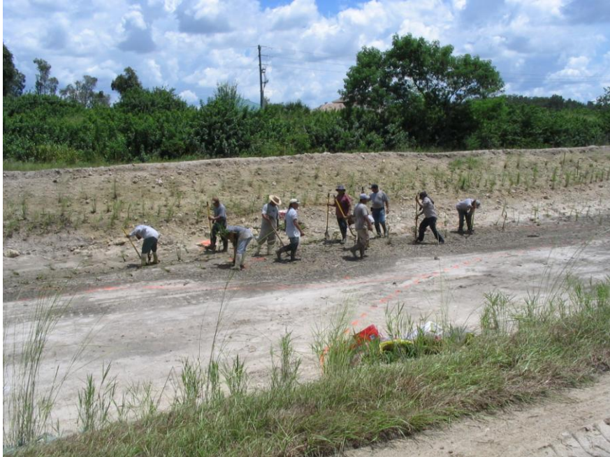
August 24, 2005 Emergent wetland plants being installed by hand.
