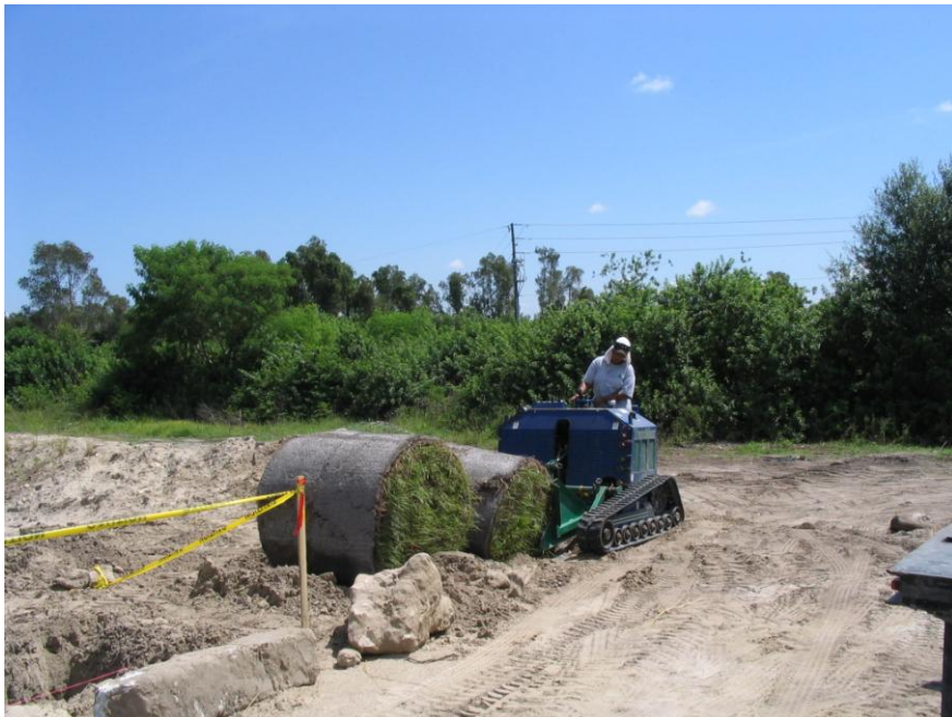
August 18, 2005 Laying sod on side slopes (typical) to stabilize excavation.
