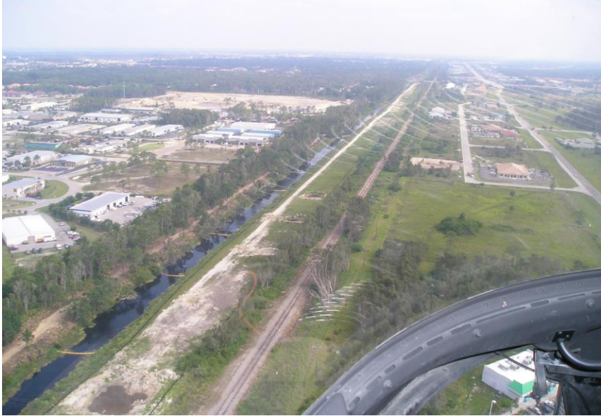
May 13, 2005 Preconstruction view from south to north.
