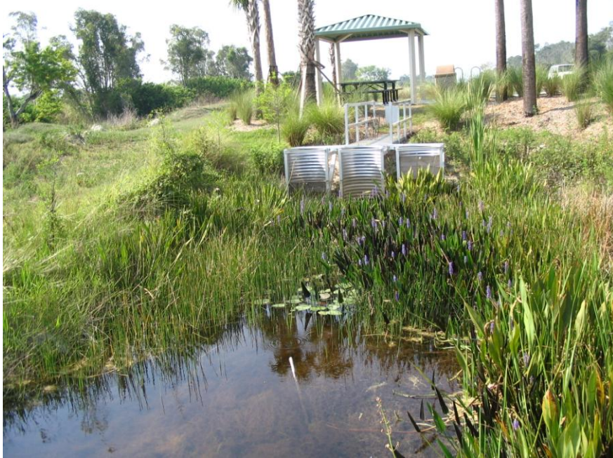
October 24, 2005 The control structure connecting Cell No. 2 to Cell No. 3. Looking south. The maintenance ramp to Cell No.2 is on the left.
