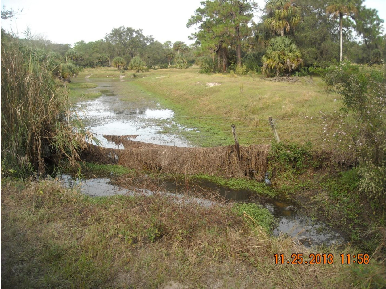
Fence Covered in debris
